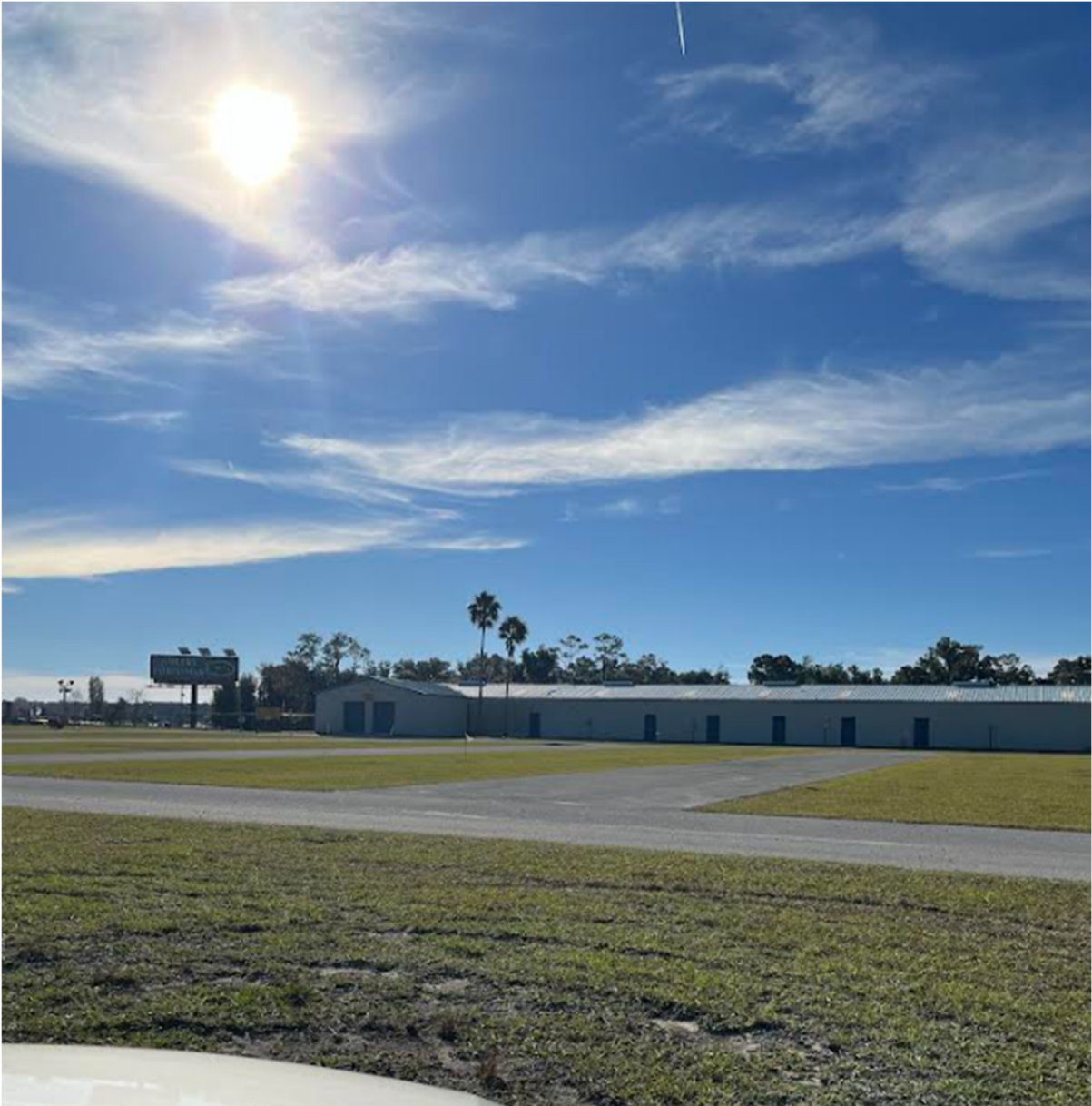
Pond B11C, B12C & B13A (A-2) 4121 NW 44 th Avenue (North Side)
