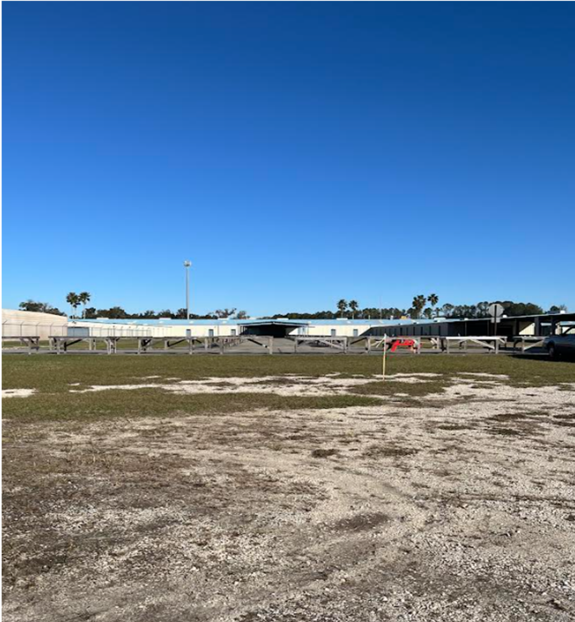
Pond B11C, B12C & B13A (A-2) 4121 NW 44 th Avenue (South Side)
