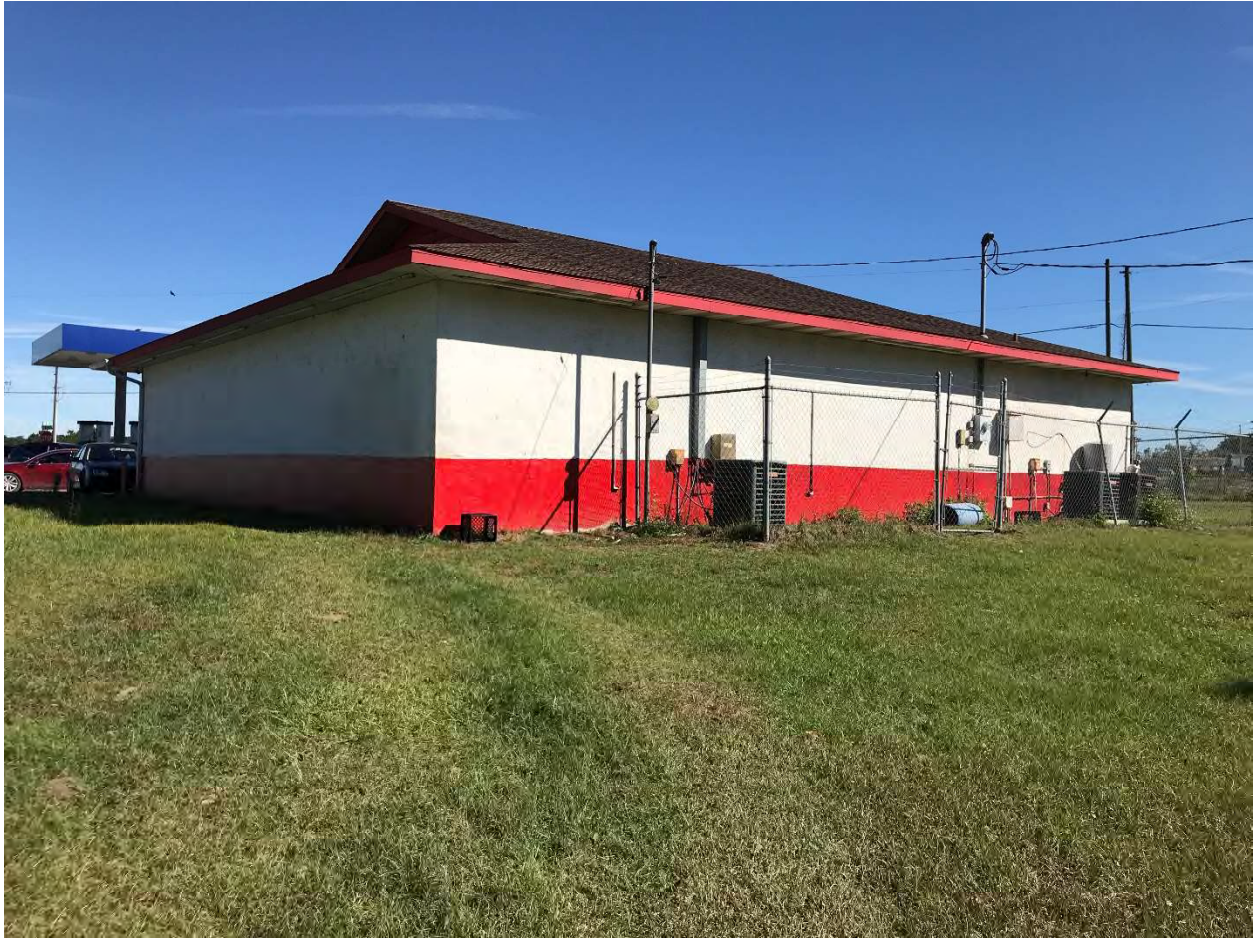
Rear of Building, Facing Northeast
