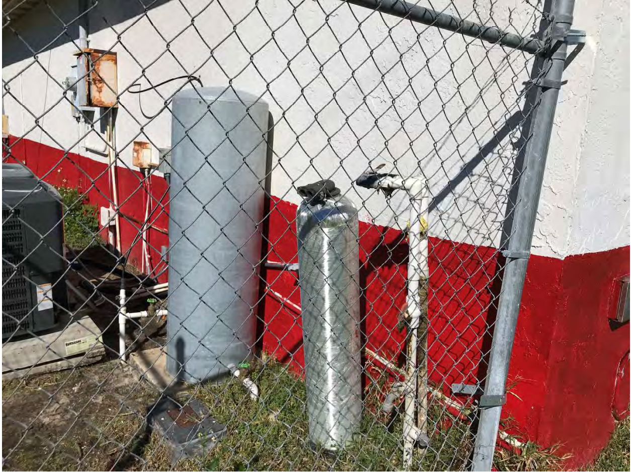
Tanks at Rear of Building
