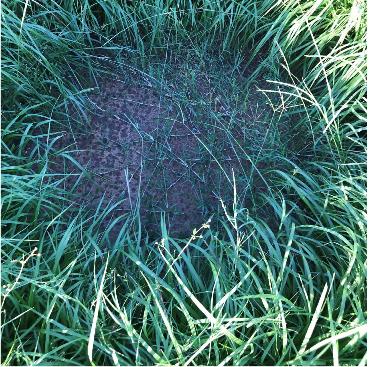
Water Filled Hole Surrounded by Barriers
