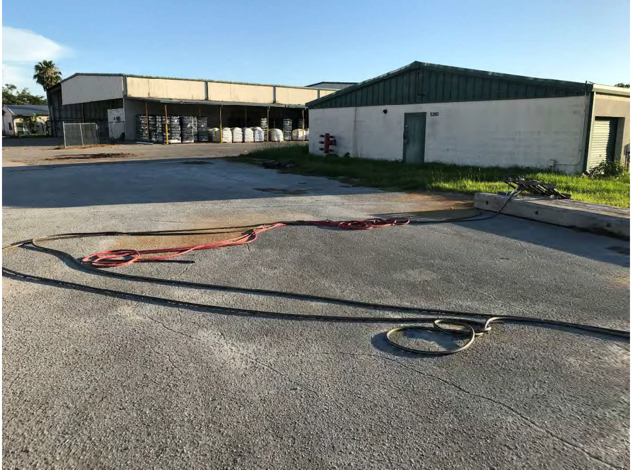
Possible Truck Wash Down Area, Facing Southwest
