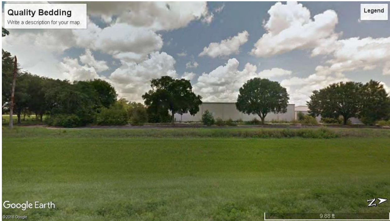
View of Quality Bedding, Facing West From I-75
