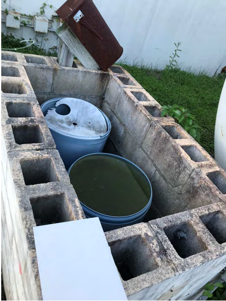
Open Drums Beside AST
