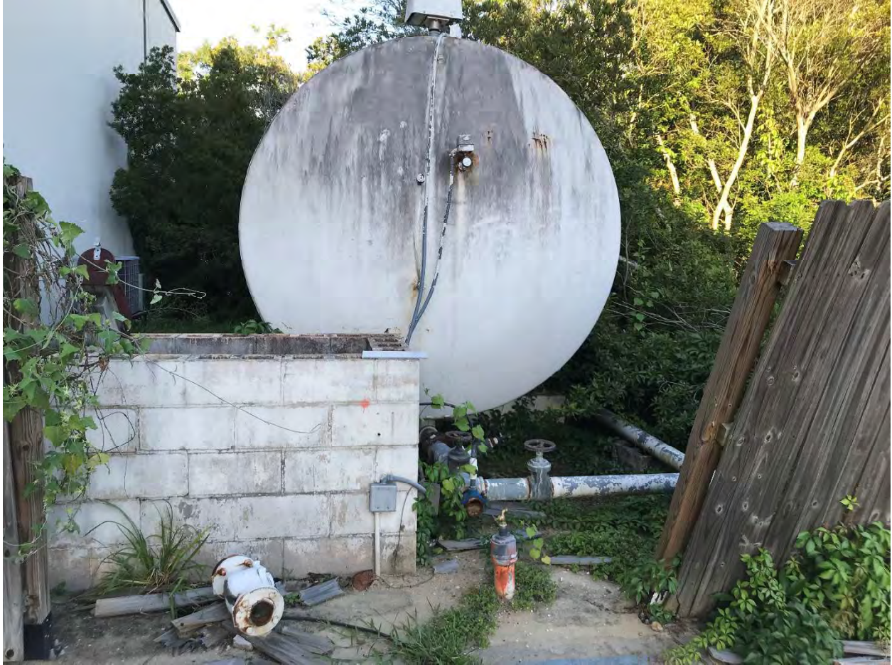
AST on South Side of Quality Bedding Building, Facing East
