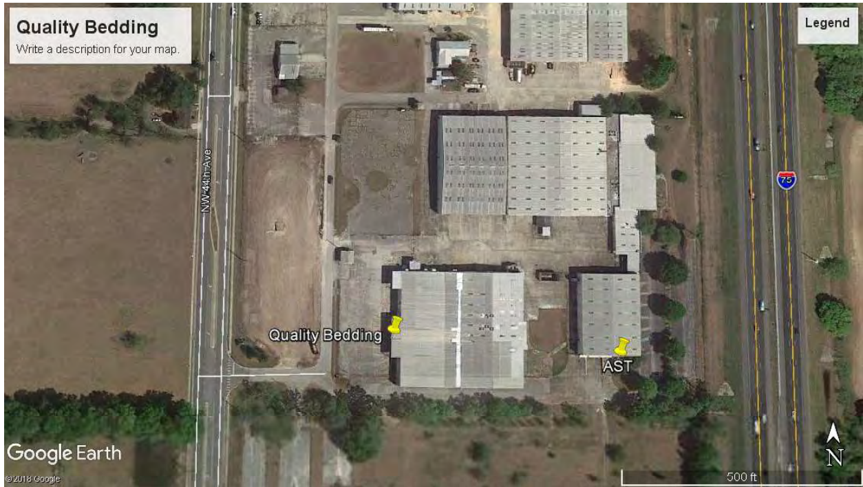
Hydro Spa/Quality Bedding Aerial View
