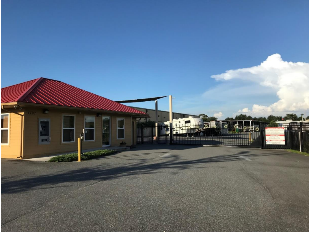
Photograph 5-1 Barracuda Boat and RV Storage Entrance, facing east
