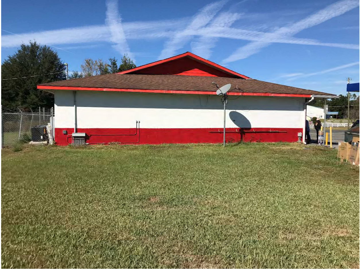
Side of Building, Facing North
