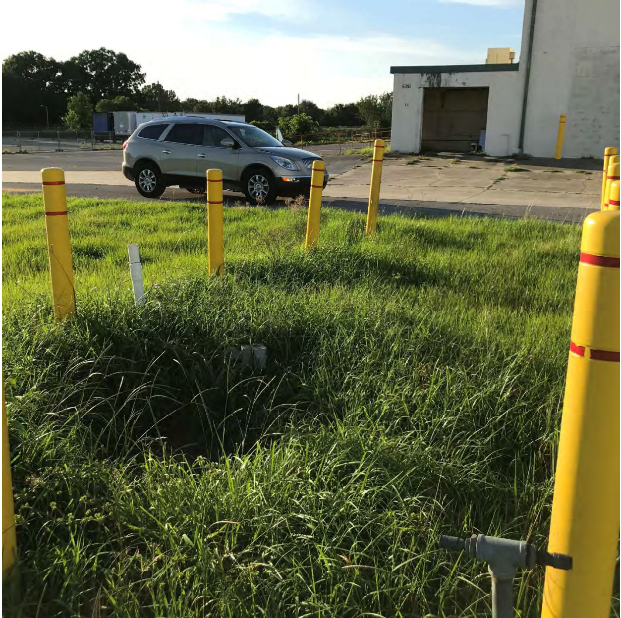
Barriers around water feature, facing north
