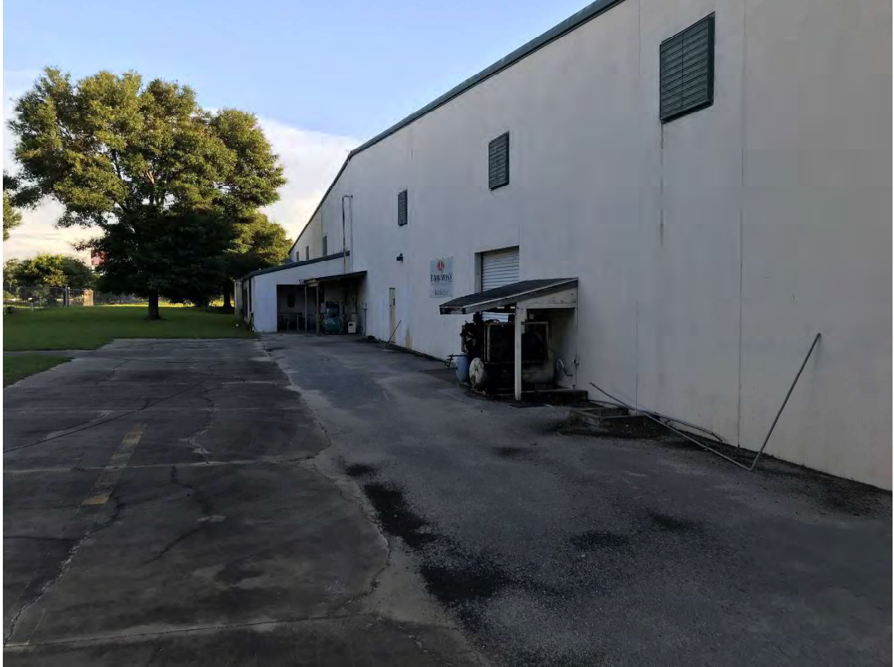
ASTs on East Side of Hickory Springs Buildings, Facing South
