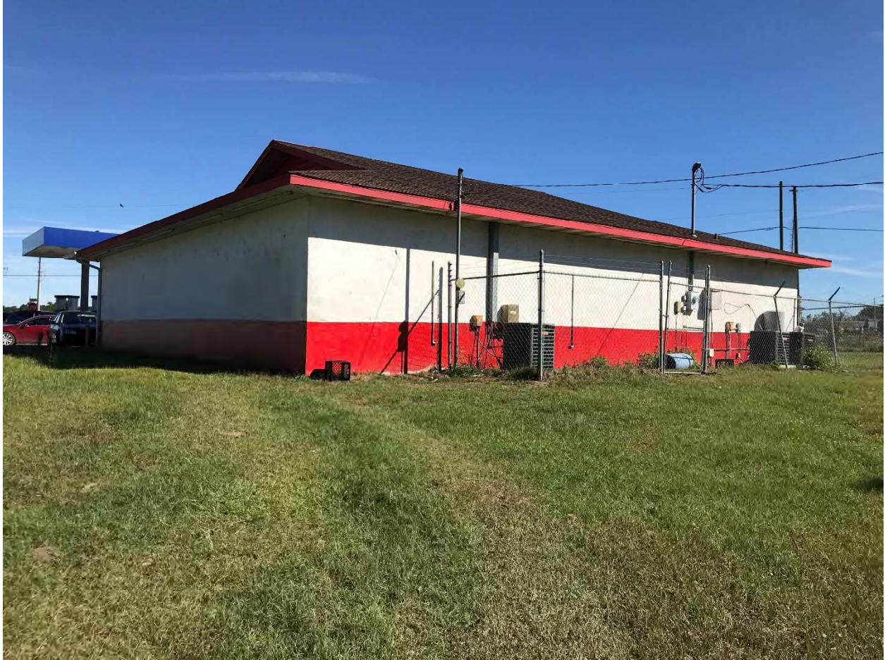
Rear of Building, Facing Northeast
