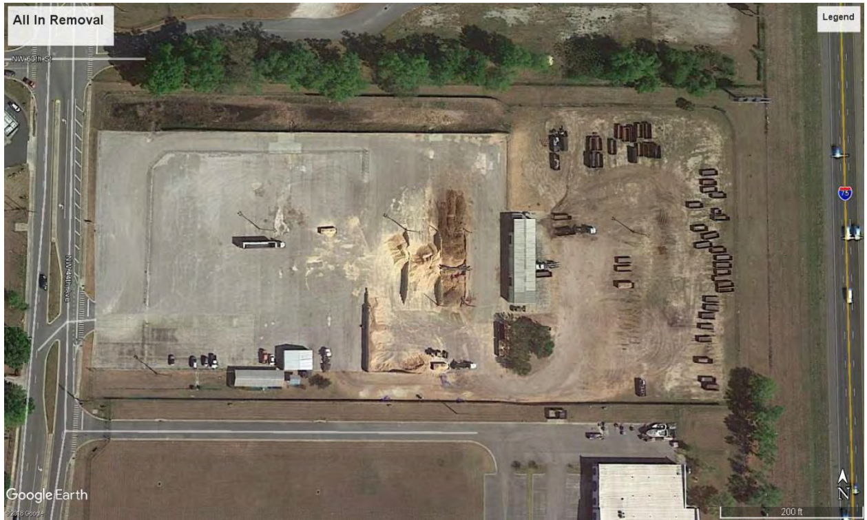
Aerial View of All In Removal
