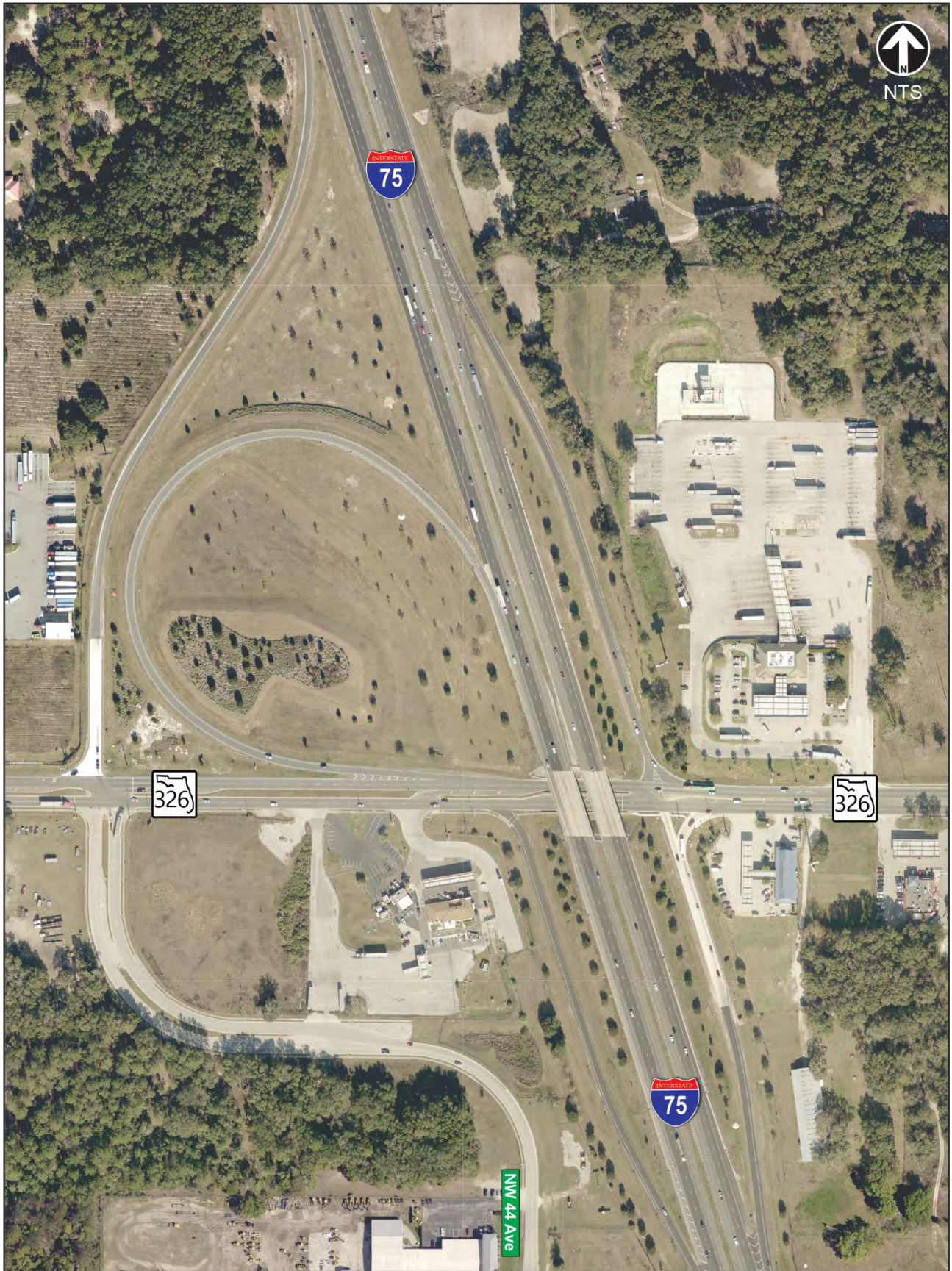
Figure 3-2: I-75 at SR 326 Interchange
