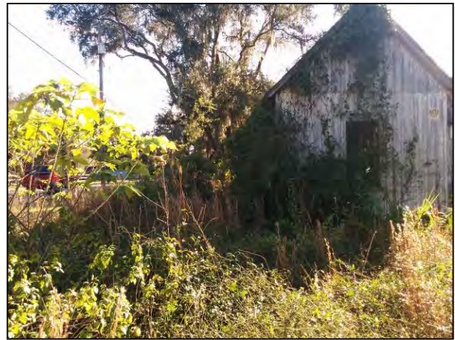
FIGURE 25 | Ca. 1930 residence (8SM00874) located south of 8SM00929, view south.
