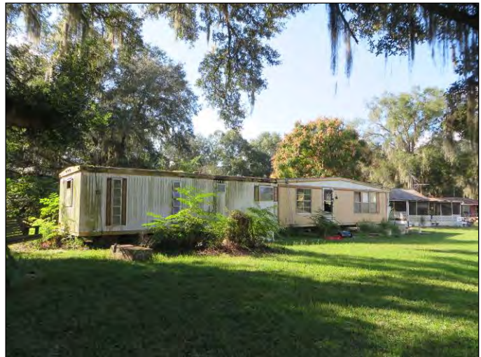
FIGURE 66 | Resource 8SM00891 is an example of a mobile home found within the US 301 PD&E APE. Photograph facing northwest.
