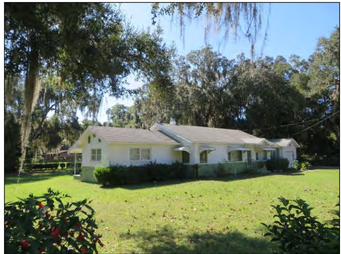
FIGURE 60 | Resource 8SM00843 is an example of a Ranch style building found within the US 301 PD&E APE. Photograph facing southwest.
