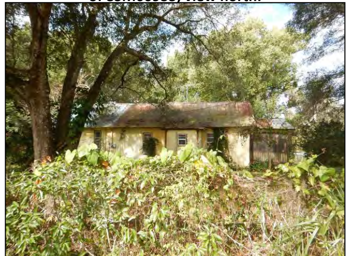
FIGURE 46 | Ca. 1955 residence located north of 8SM00935, view north.
