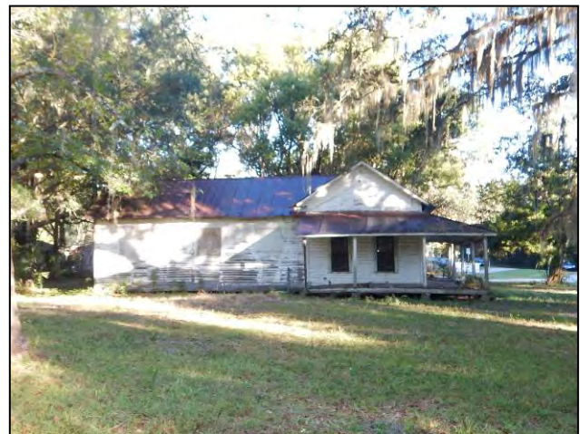
FIGURE 29 | Ca. 1920 historic residence (8SM00883) located north of 8SM00930, view north.
