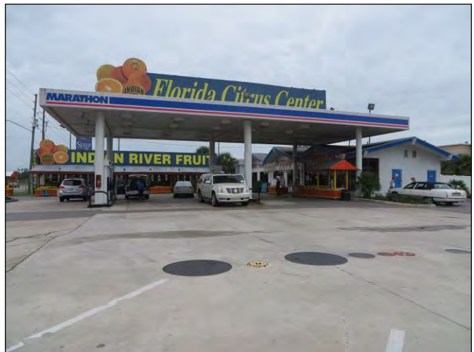
FIGURE 61 | Resource 8SM00801 is an example of a Commercial style building found within the US 301 PD&E APE. Photograph facing north.
