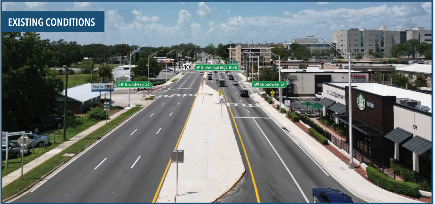
Existing conditions on the northbound South Pine Avenue approach to the intersection with West Silver Springs Boulevard.
