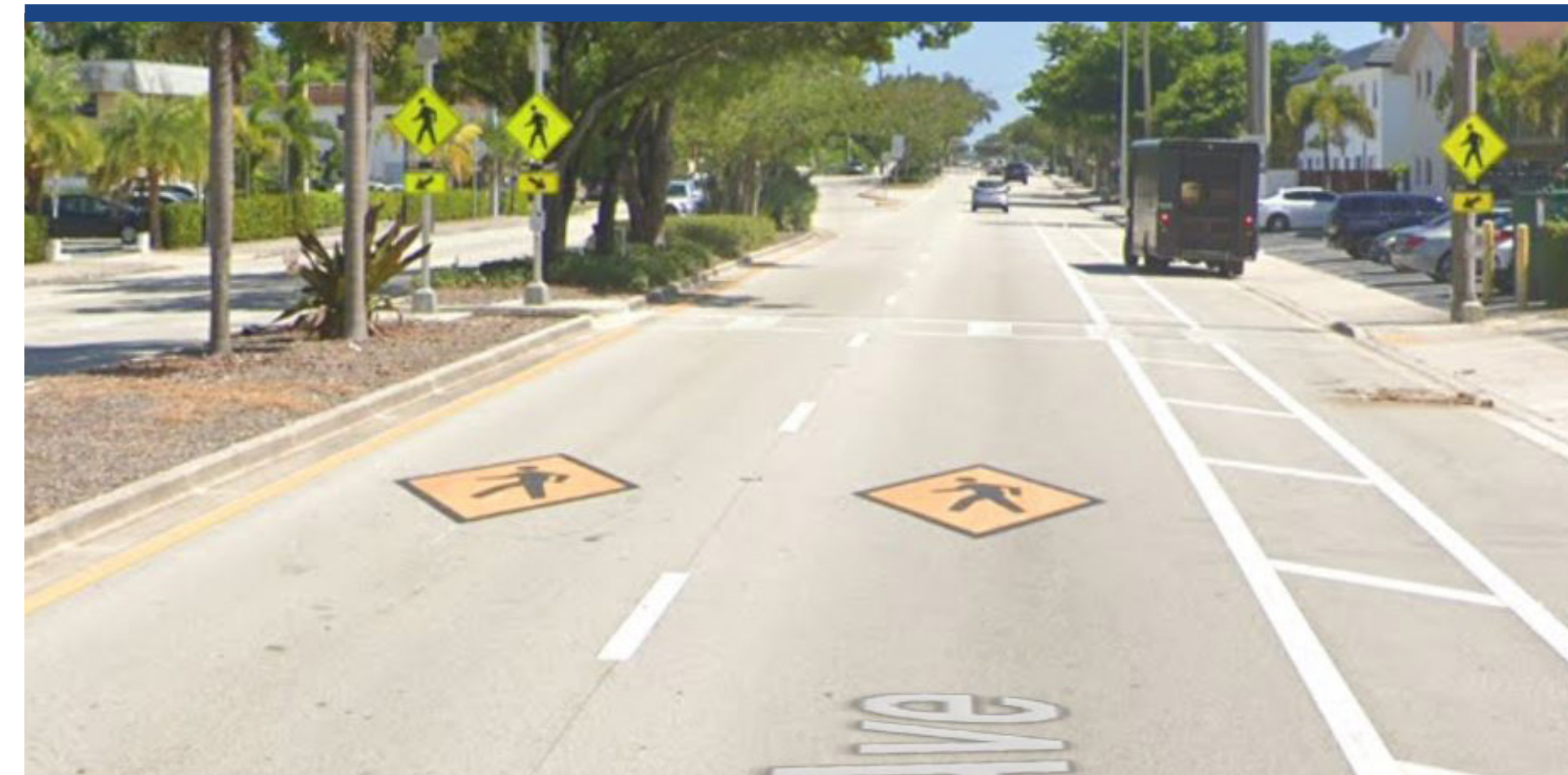
▼ Thermoplastic Decal on Roadway
