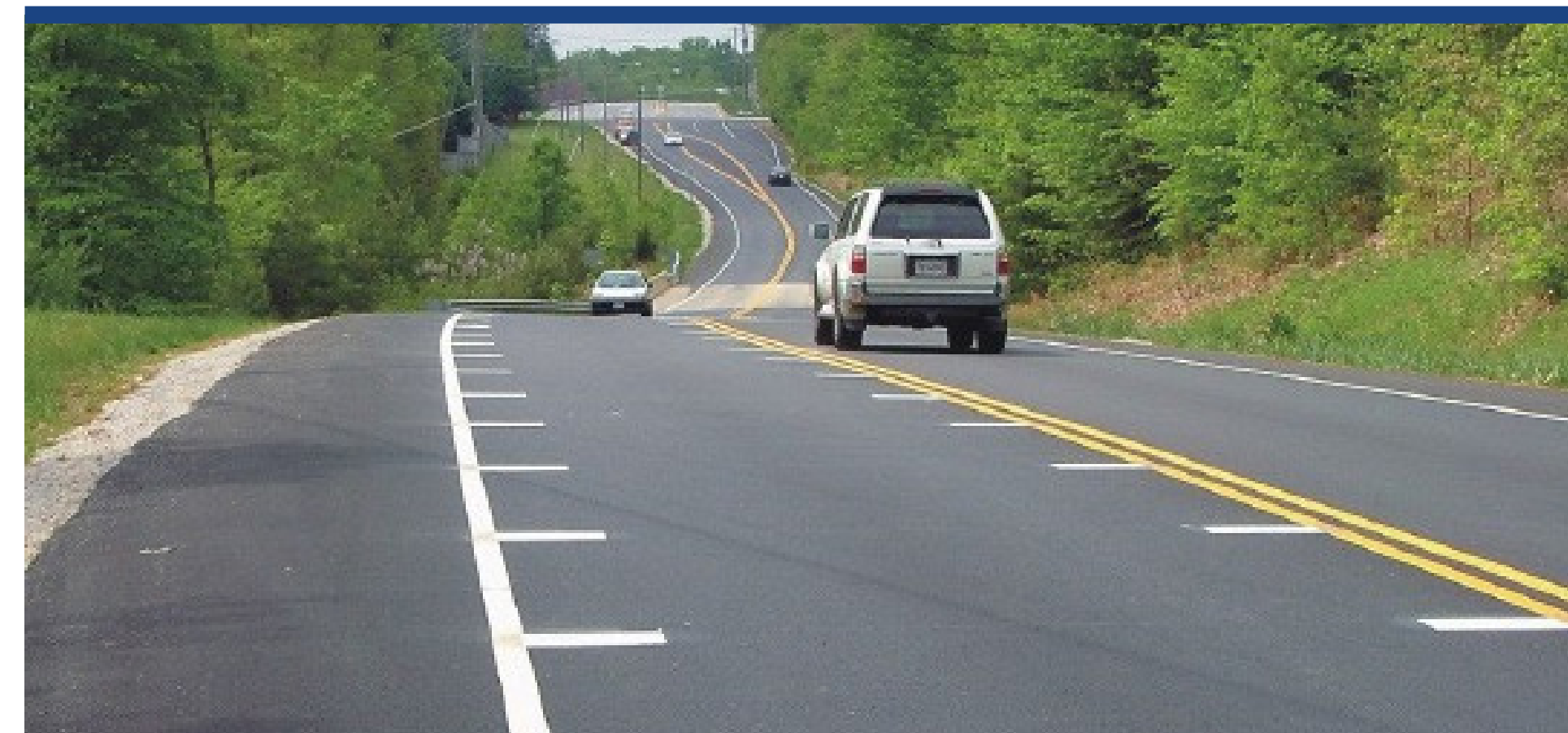
▼ Thermoplastic Decal on Roadway
