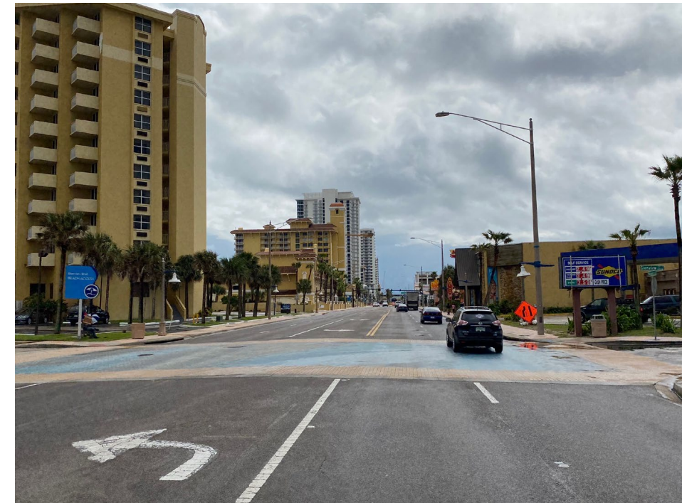
Lack of safe crossings
