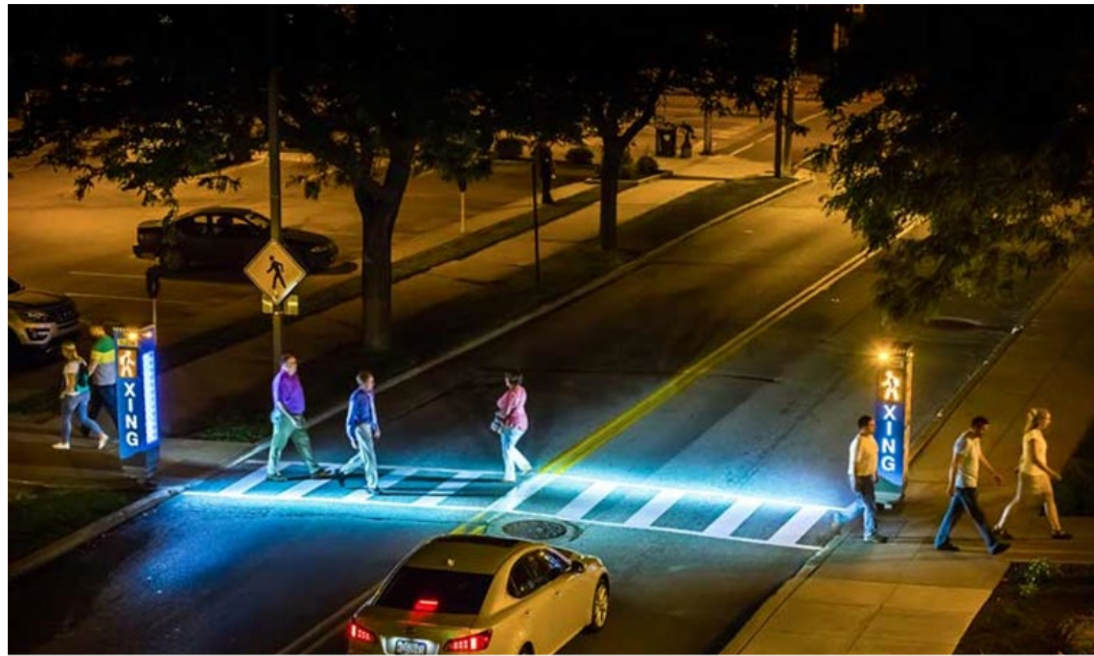
High Emphasis Pedestrian Crosswalk Lighting
