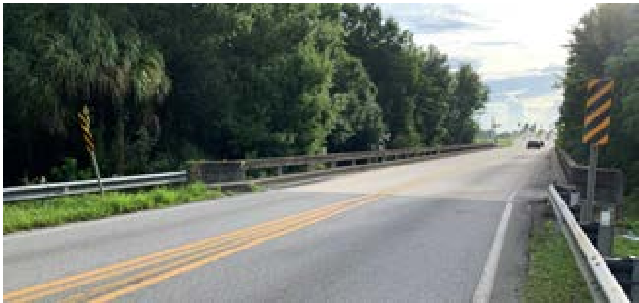
Figure 2.9 | Bridge No. 794038 West Approach
