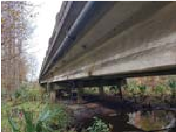
Figure 2.10 | South Elevation, Span 5
