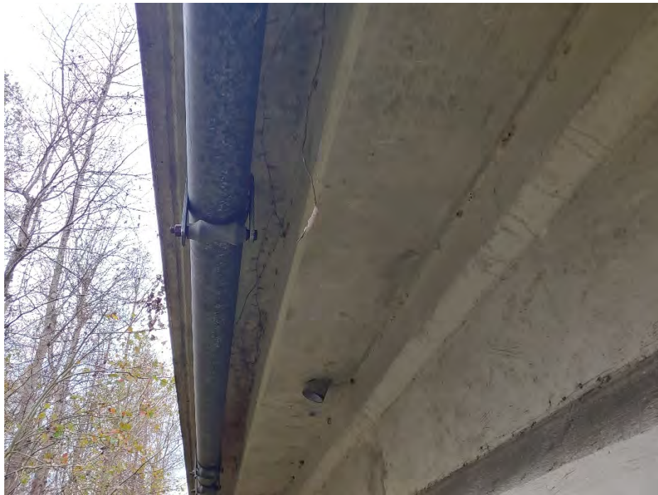
Scupper and utility pipe
