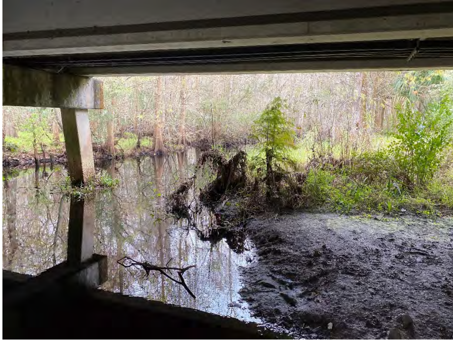
Looking south under the bridge
