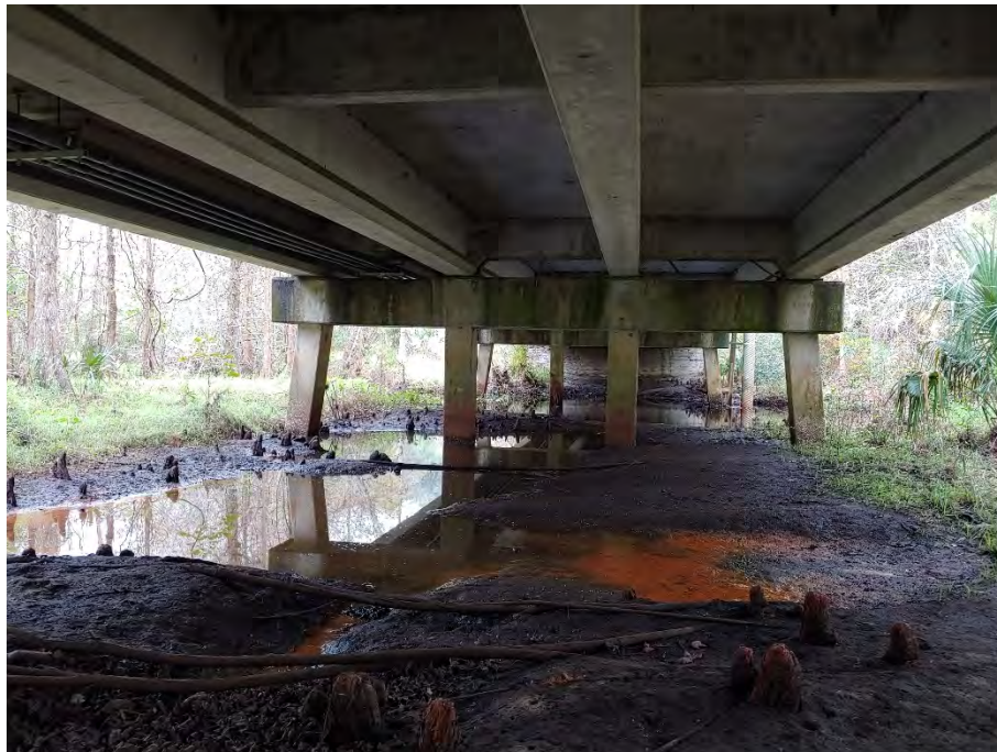
Looking west under the bridge
