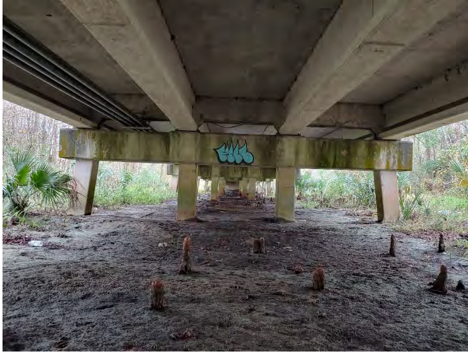
Looking east under the bridge
