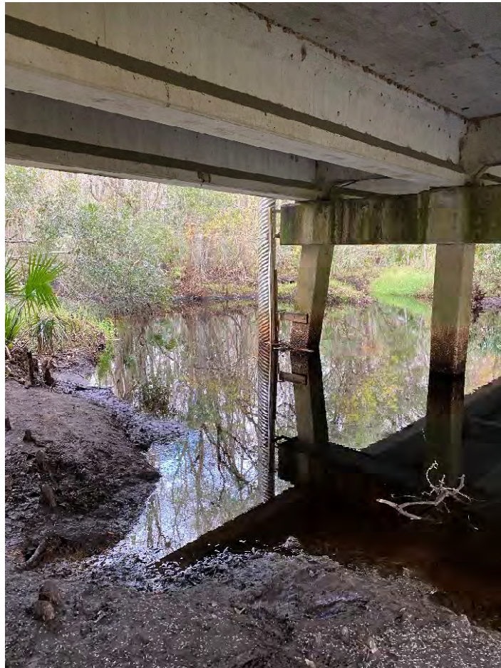
Looking north under the bridge
