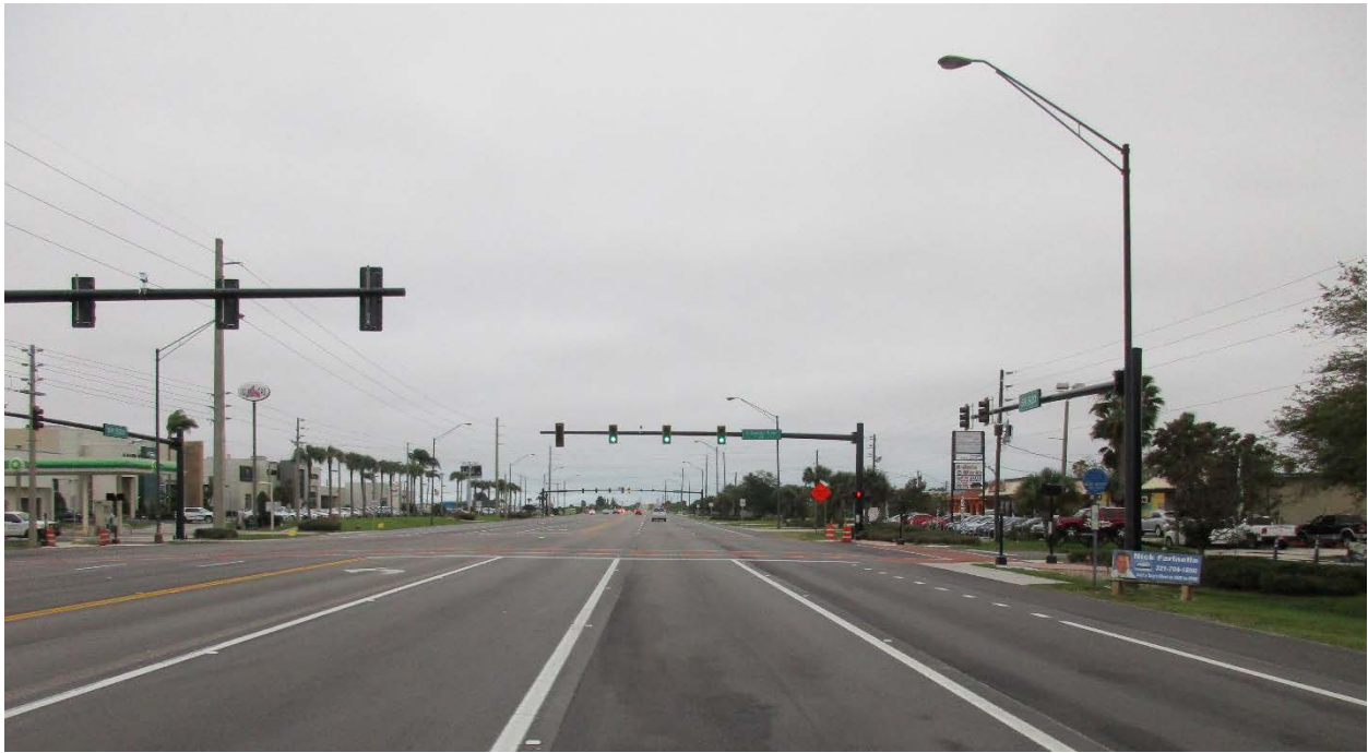
Looking East along SR 520 at the North Banana River Drive Intersection
