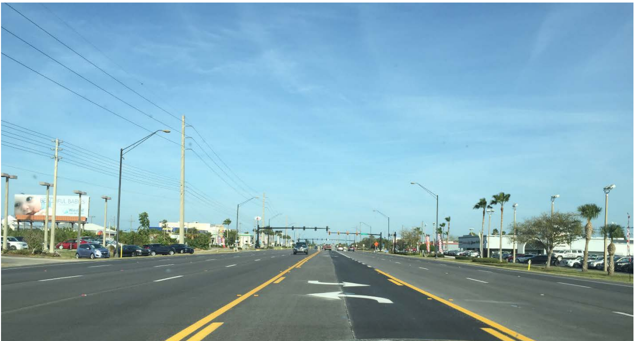
Looking East at the Two-Way Left Turn Lane along SR 520
