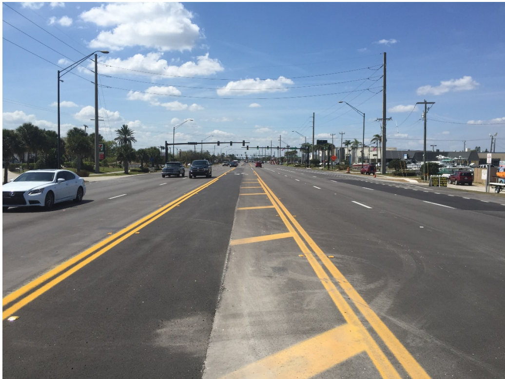
Looking West along SR 520 at the End of Study Limits
