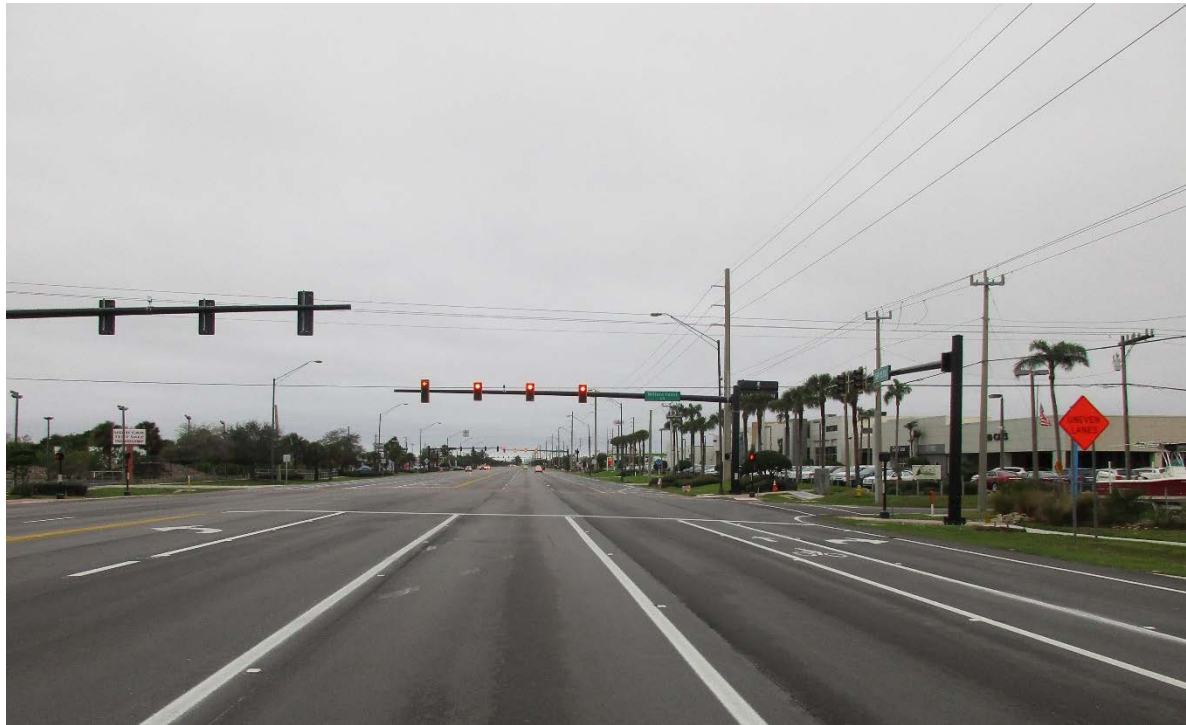
Looking West along SR 520 at the South Banana River Drive Intersection
