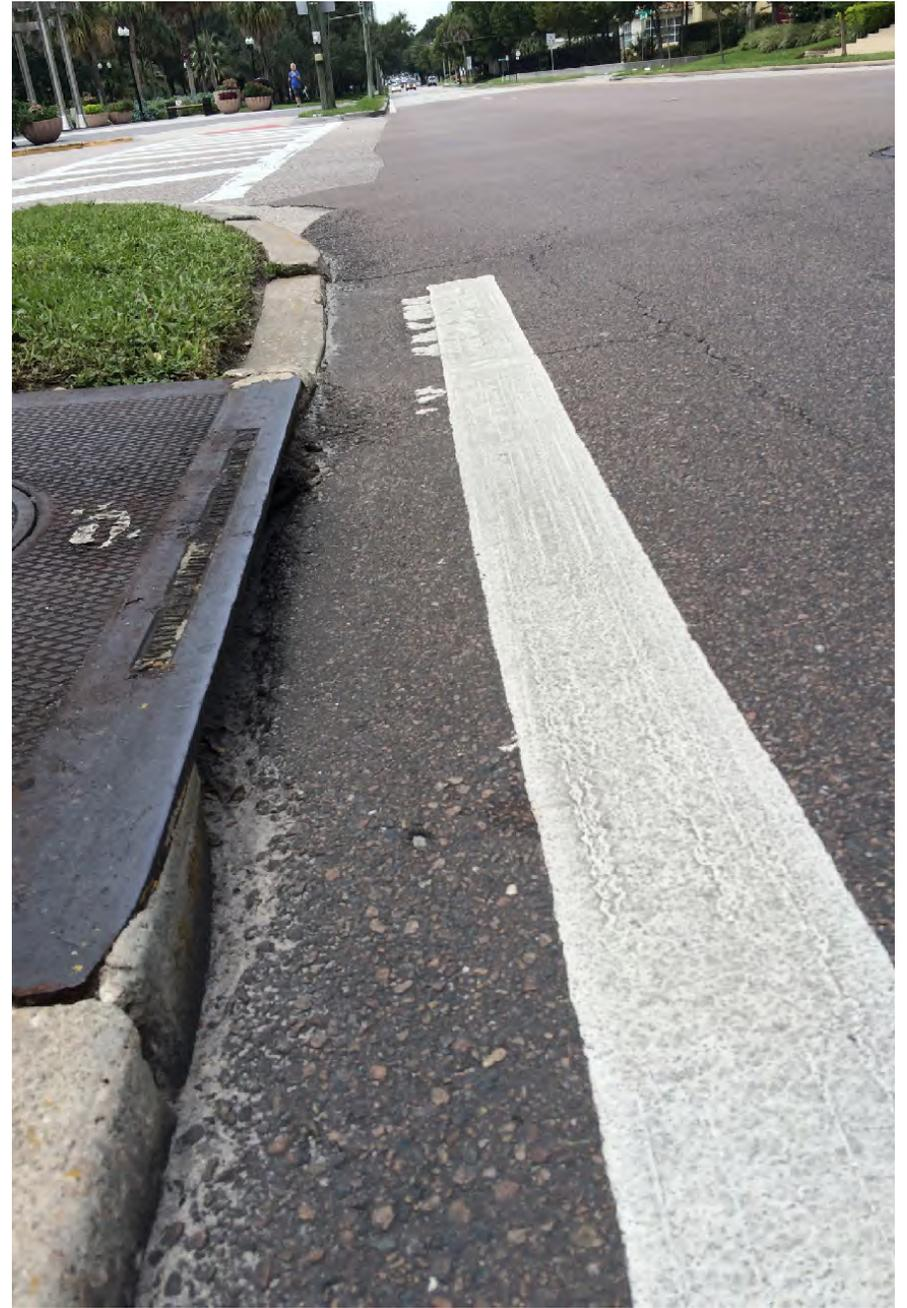
*High asphalt restricts flow at some drainage inlets along the corridor.*
