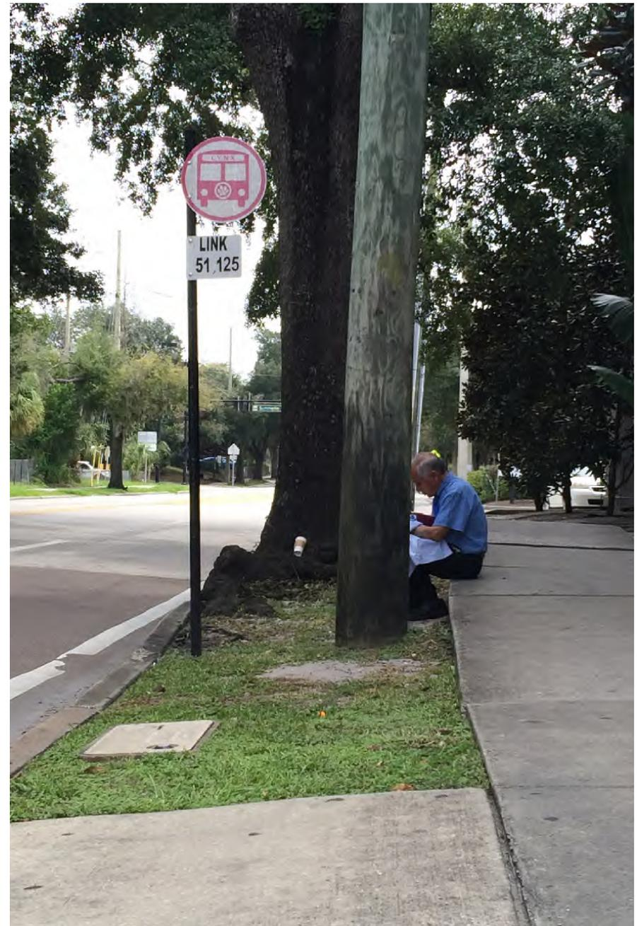
*Tree roots cause curb line to shift and sidewalks to buckle at some locations.*
