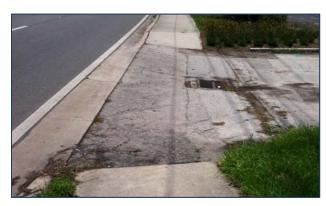
The ramps at this sidewalk lack truncated domes and the driveway has an uneven surface.
