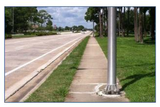
A street light reduces the usable width of the sidewalk.
