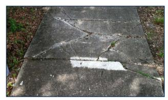
The sidewalk on Dunn Avenue, near the Nova Rd intersection, has several large cracks.
