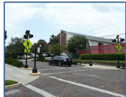
Pedestrian Signage South Ingram Avenue Lakeland, FL
