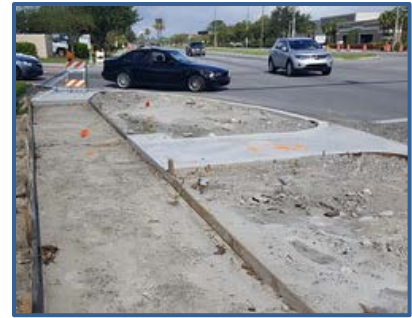
New Sidewalks US 1/Philips Highway Jacksonville, FL
