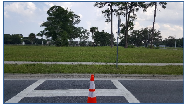
An example of a marked mid-block crossing near Chiles Academy, on George W. Engram Blvd, which lacks an ADA compliant connection.
