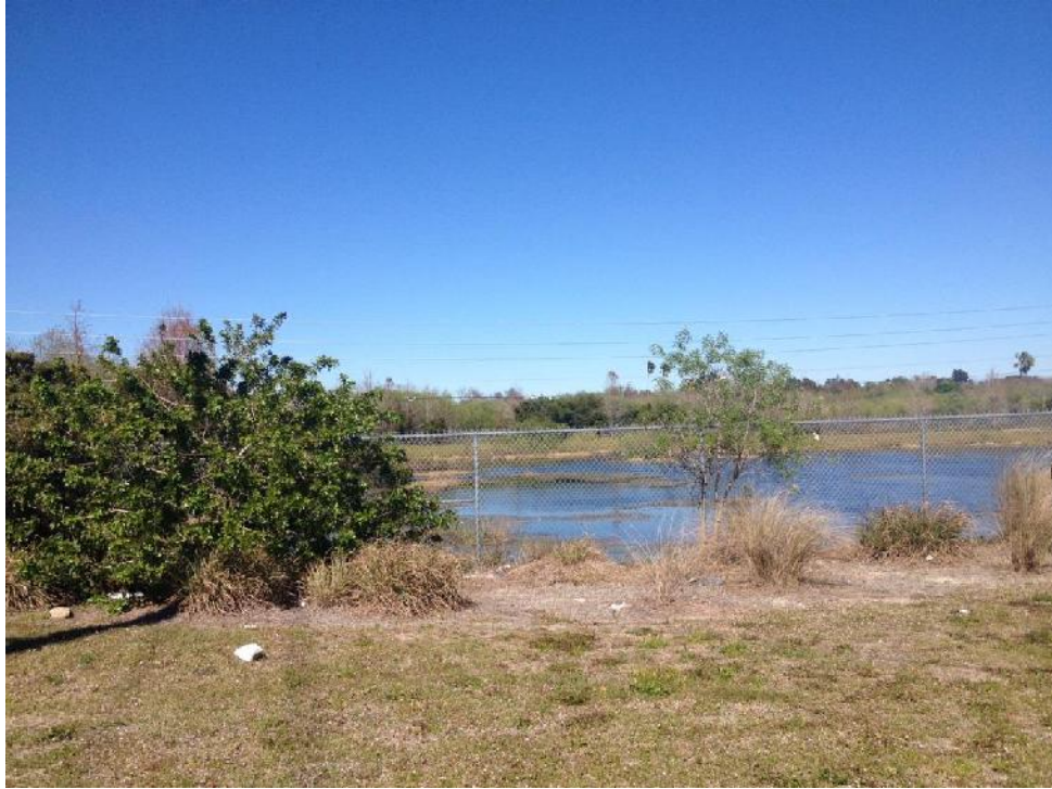
SW 1 – Stormwater Pond. View to northeast.
