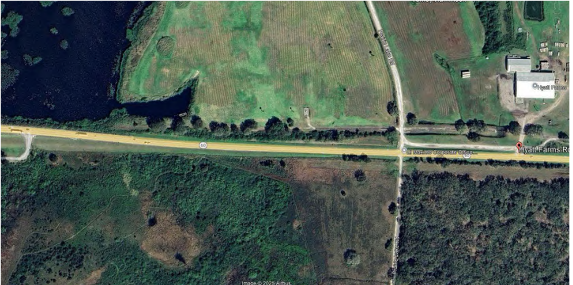
CROWN CASTLE OWNED CONDUIT VIEW
