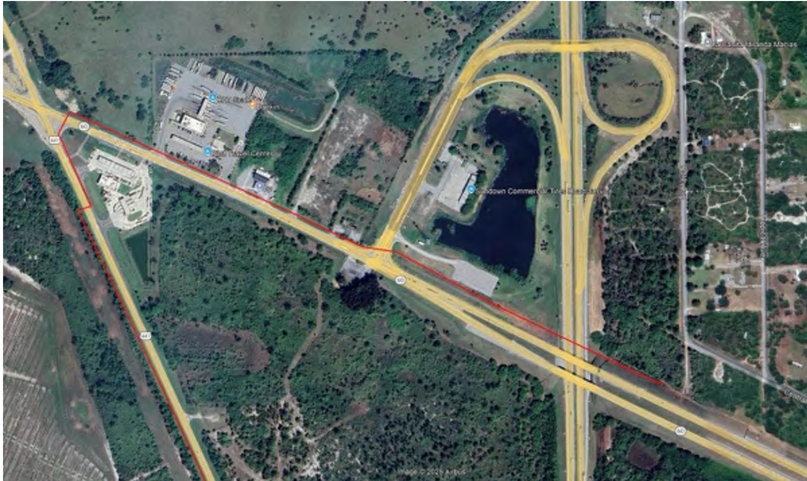
CROWN CASTLE OWNED CONDUIT VIEW
