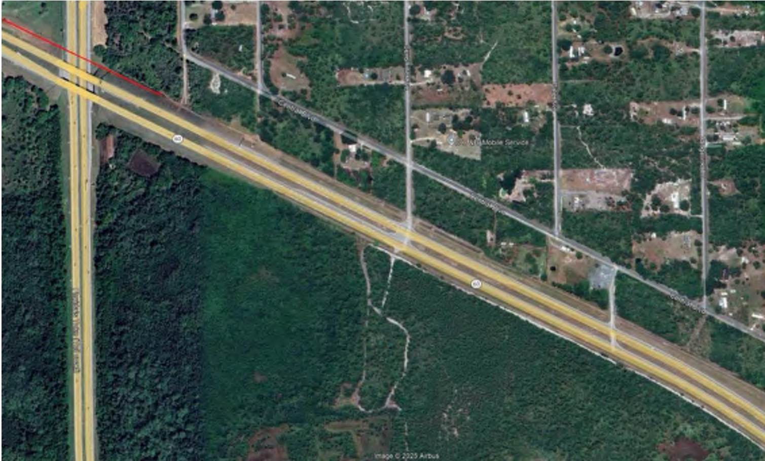
CROWN CASTLE OWNED CONDUIT VIEW
