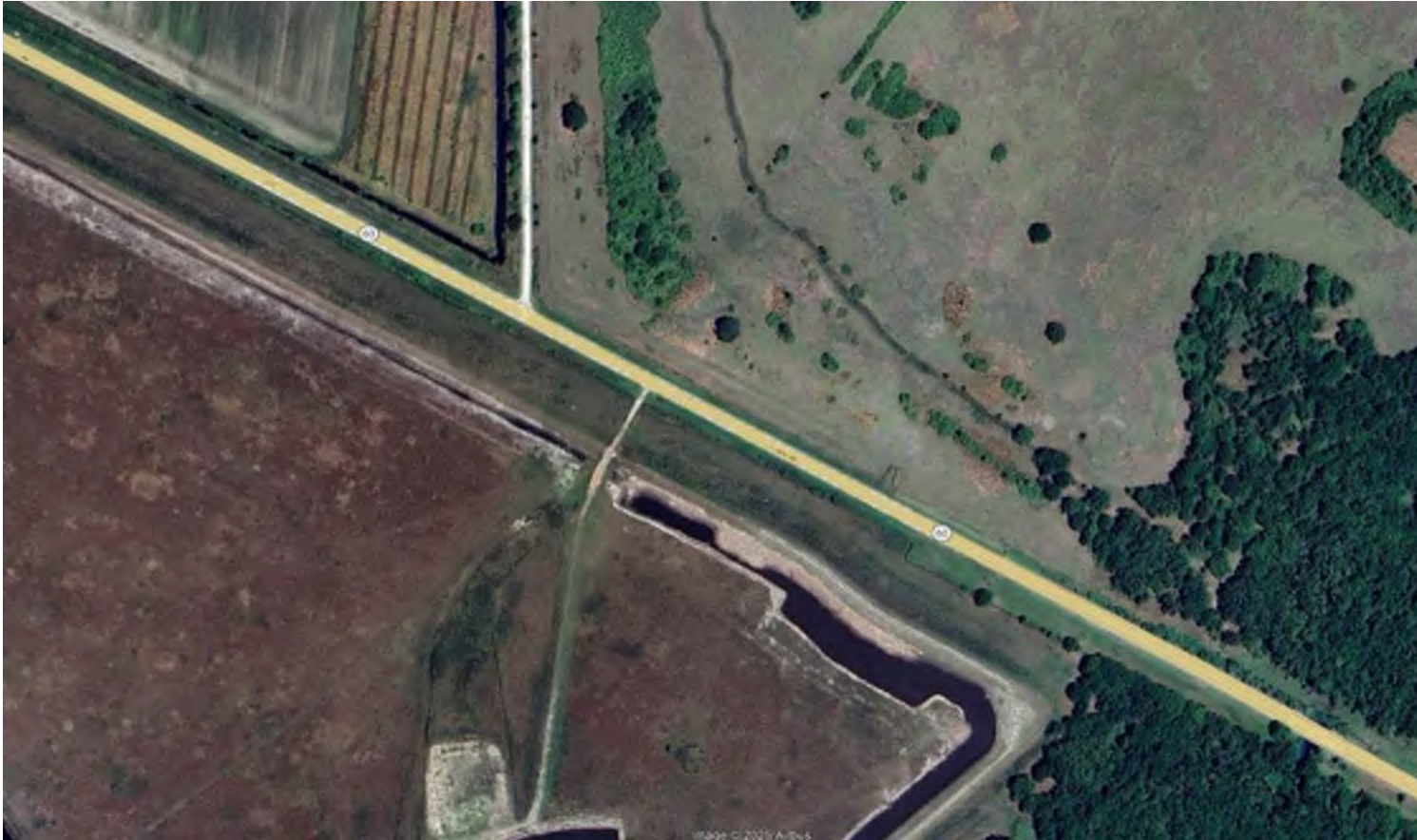
CROWN CASTLE OWNED CONDUIT VIEW
