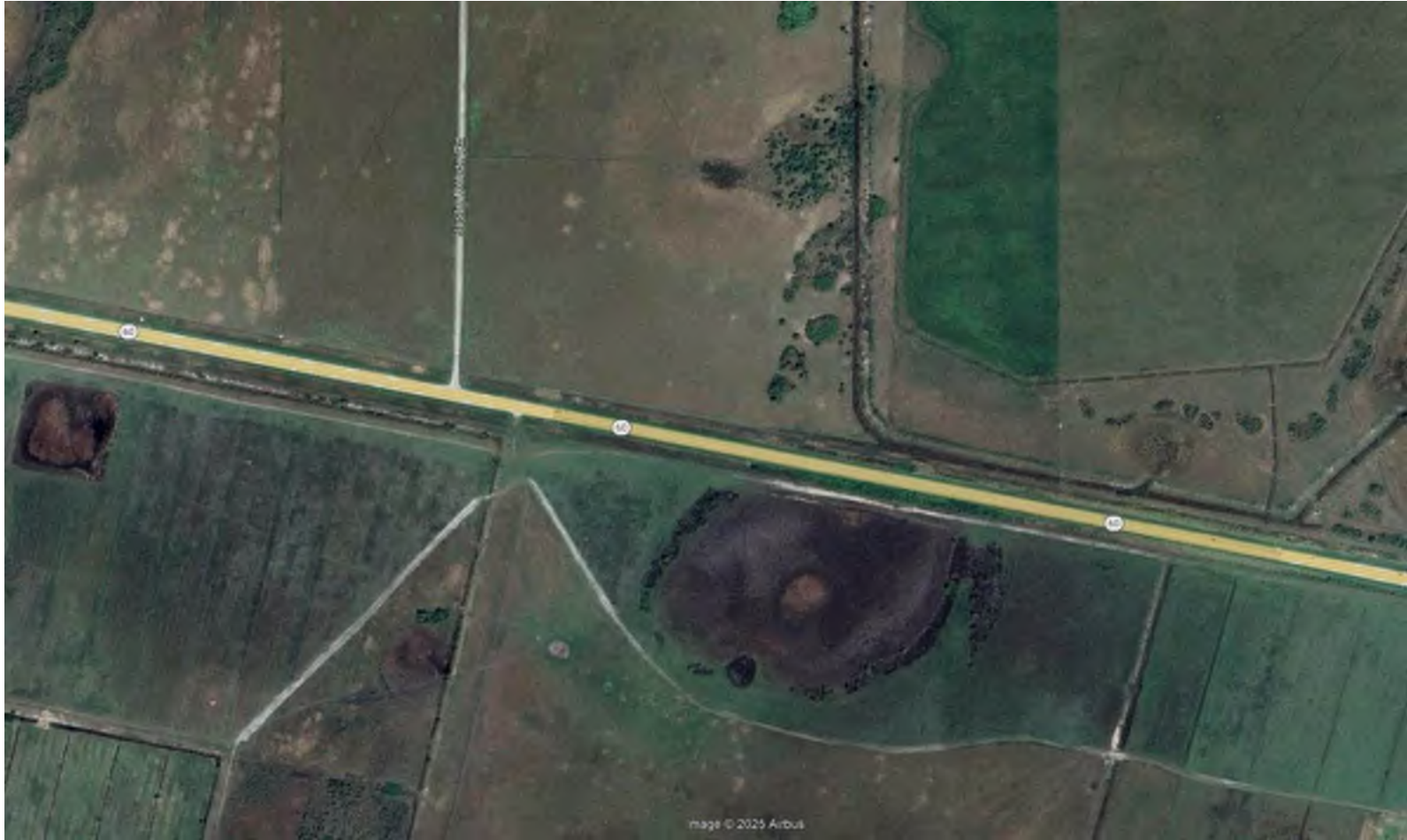
CROWN CASTLE OWNED CONDUIT VIEW
