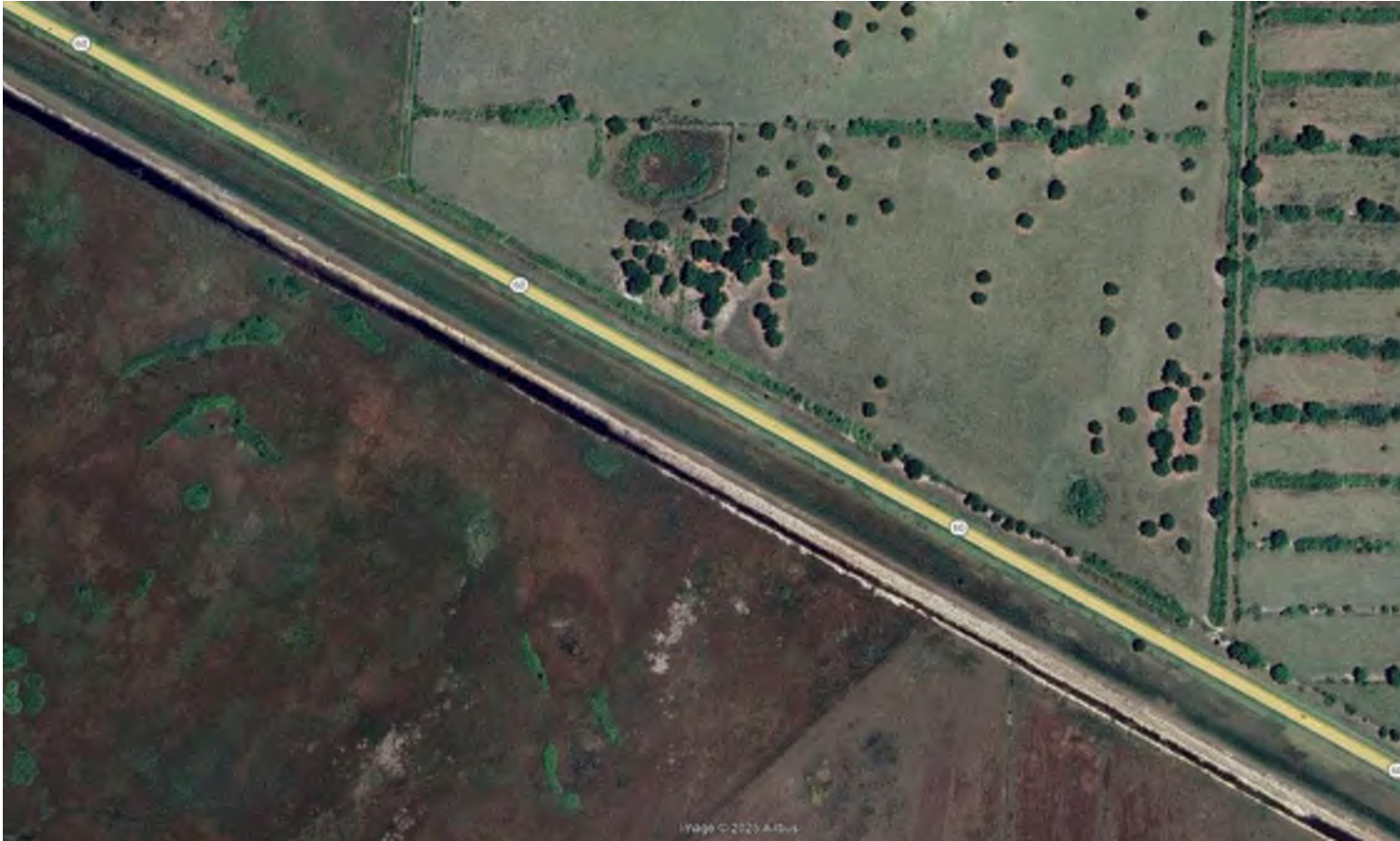
CROWN CASTLE OWNED CONDUIT VIEW
