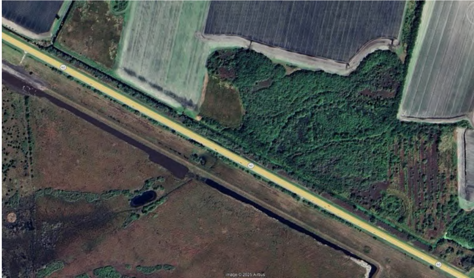
CROWN CASTLE OWNED CONDUIT VIEW
