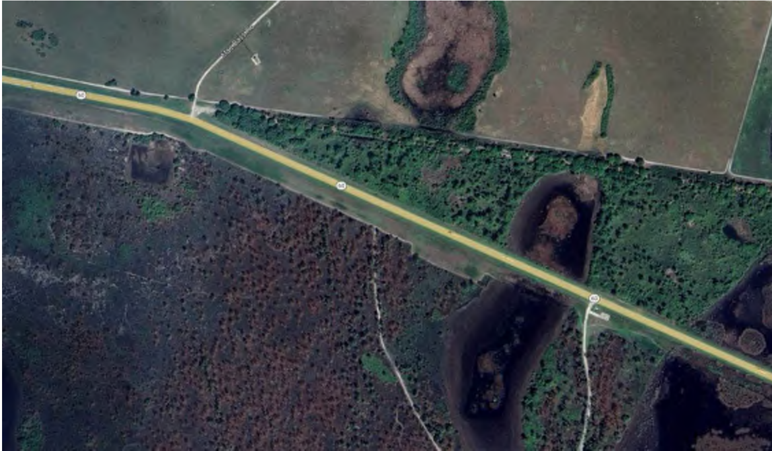
CROWN CASTLE OWNED CONDUIT VIEW
