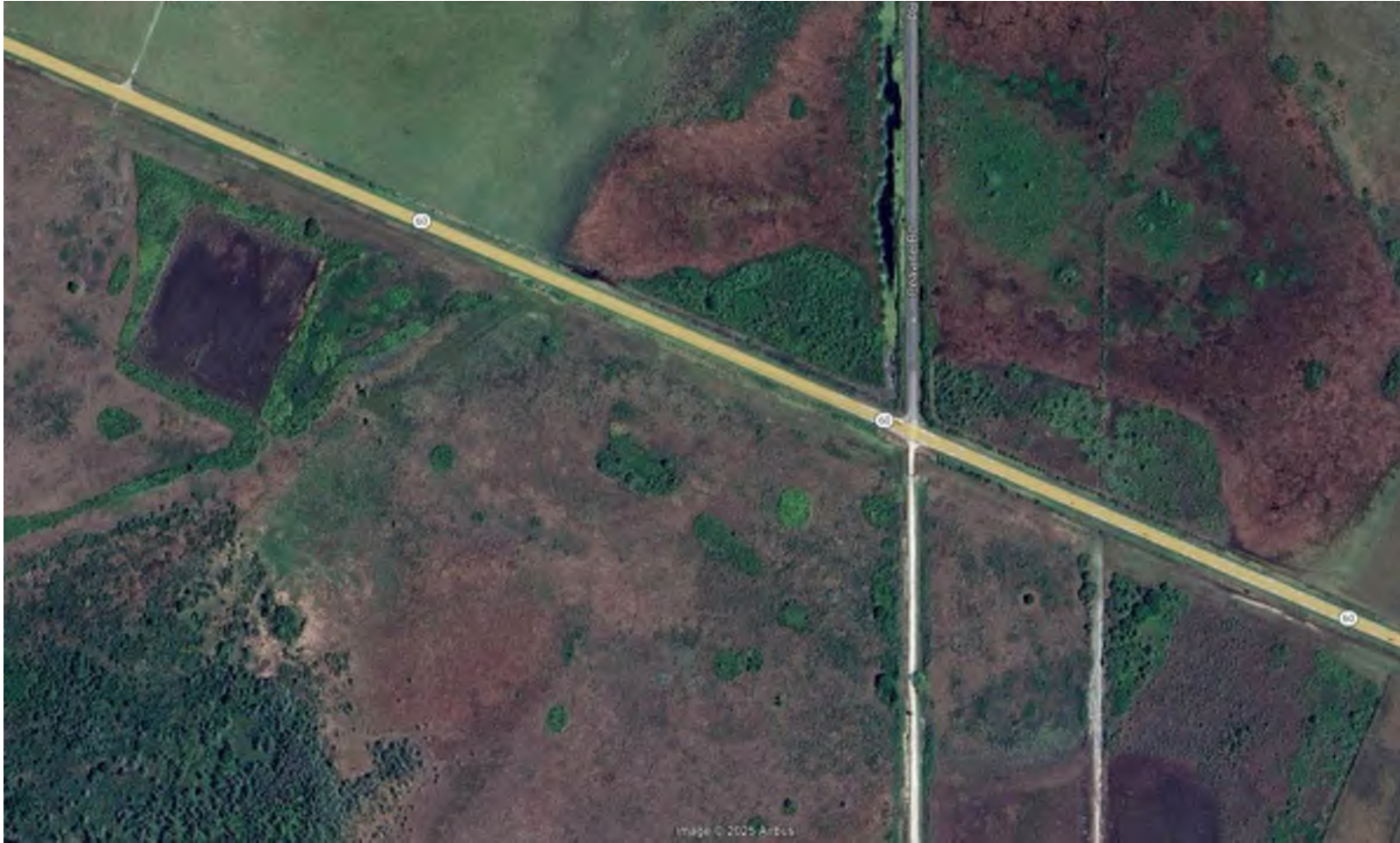
CROWN CASTLE OWNED CONDUIT VIEW
