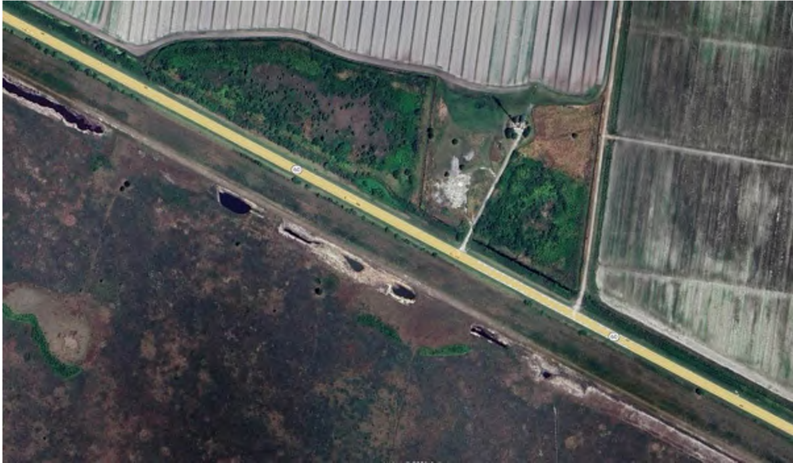
CROWN CASTLE OWNED CONDUIT VIEW
