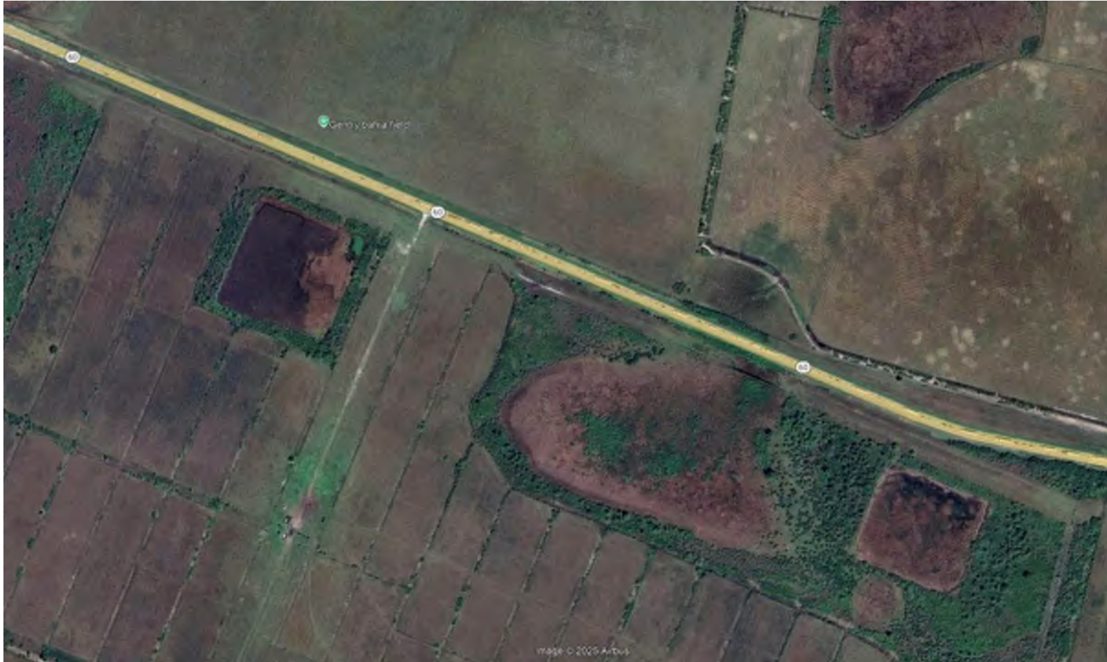
CROWN CASTLE OWNED CONDUIT VIEW
