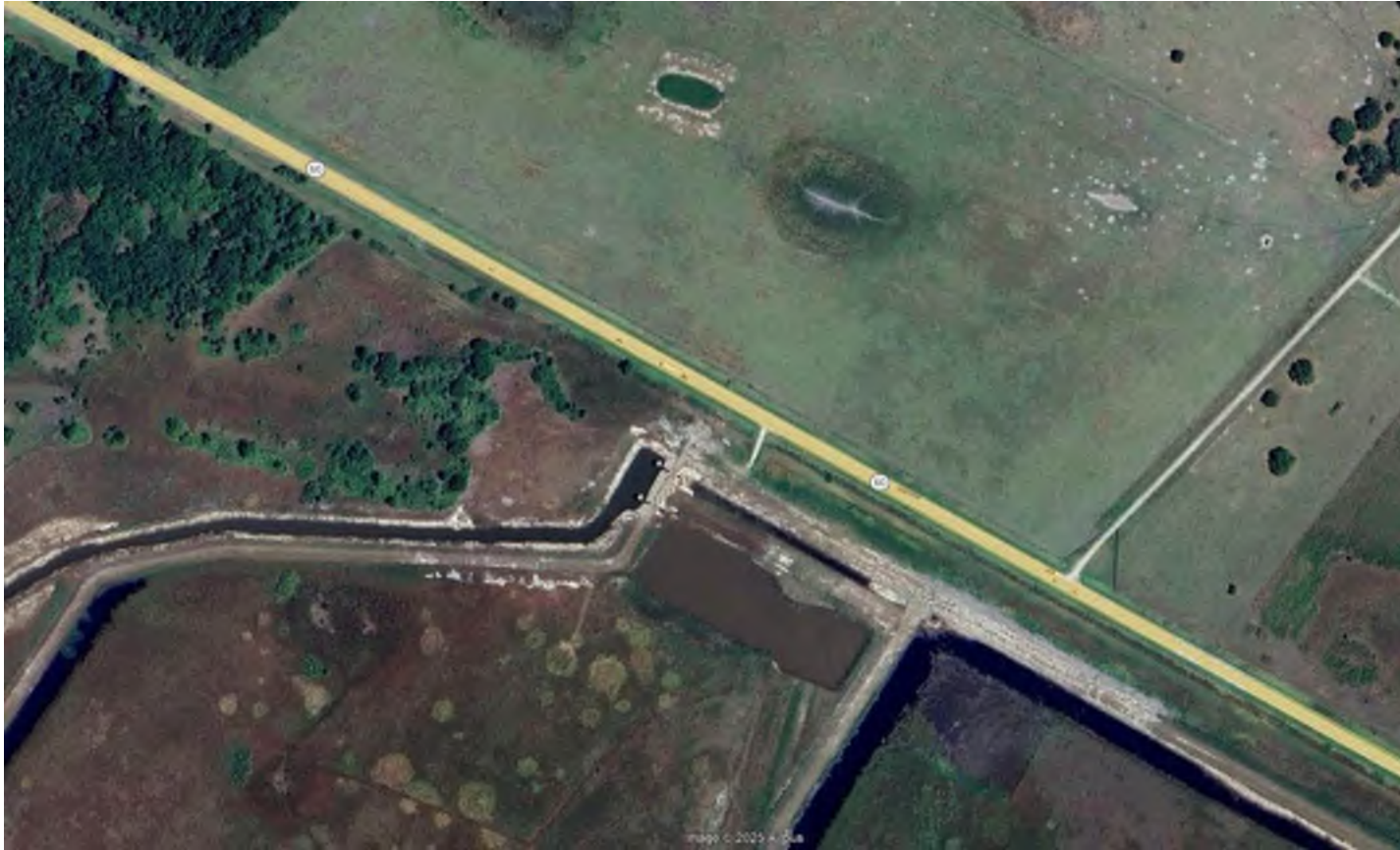
CROWN CASTLE OWNED CONDUIT VIEW
