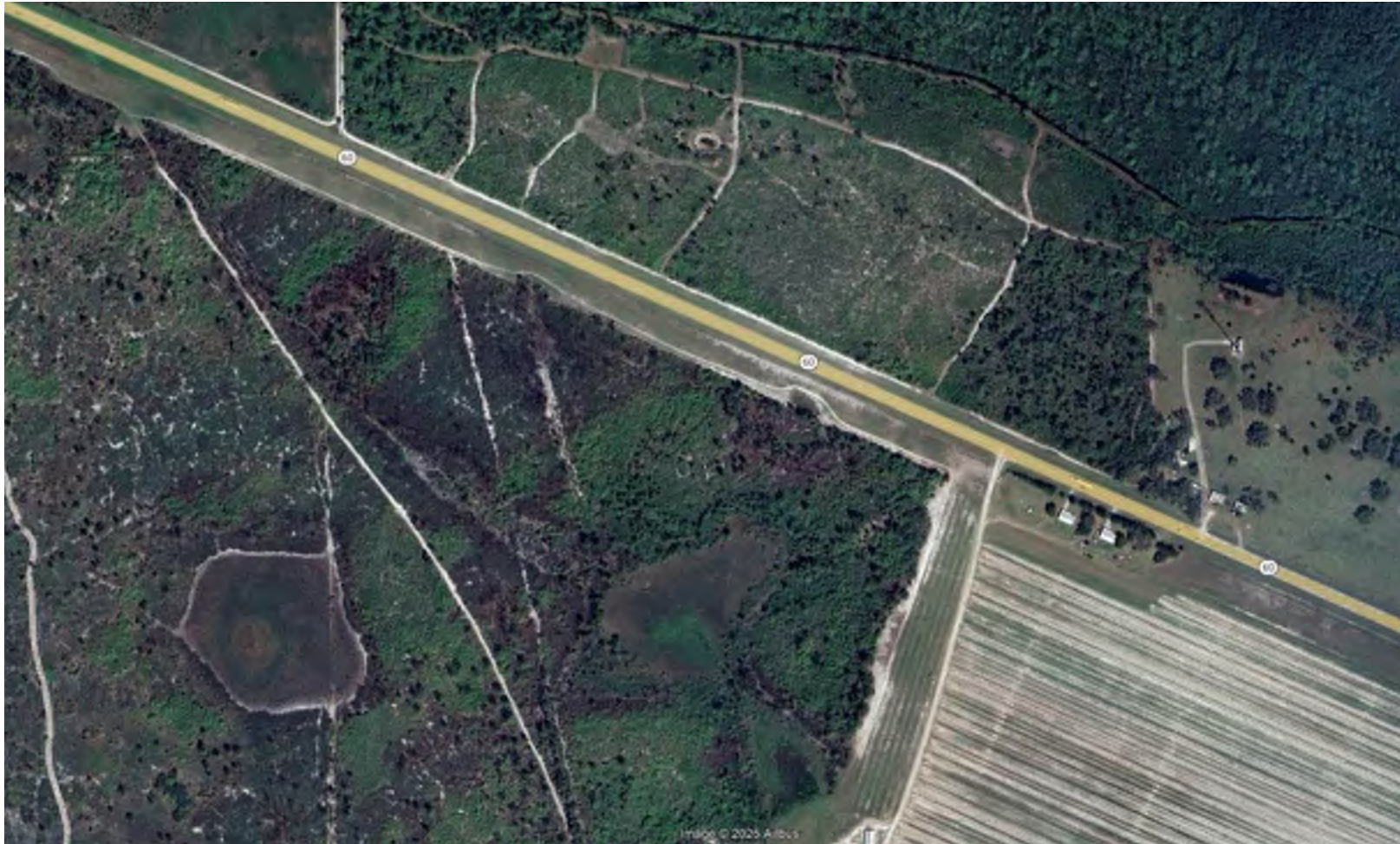
CROWN CASTLE OWNED CONDUIT VIEW
