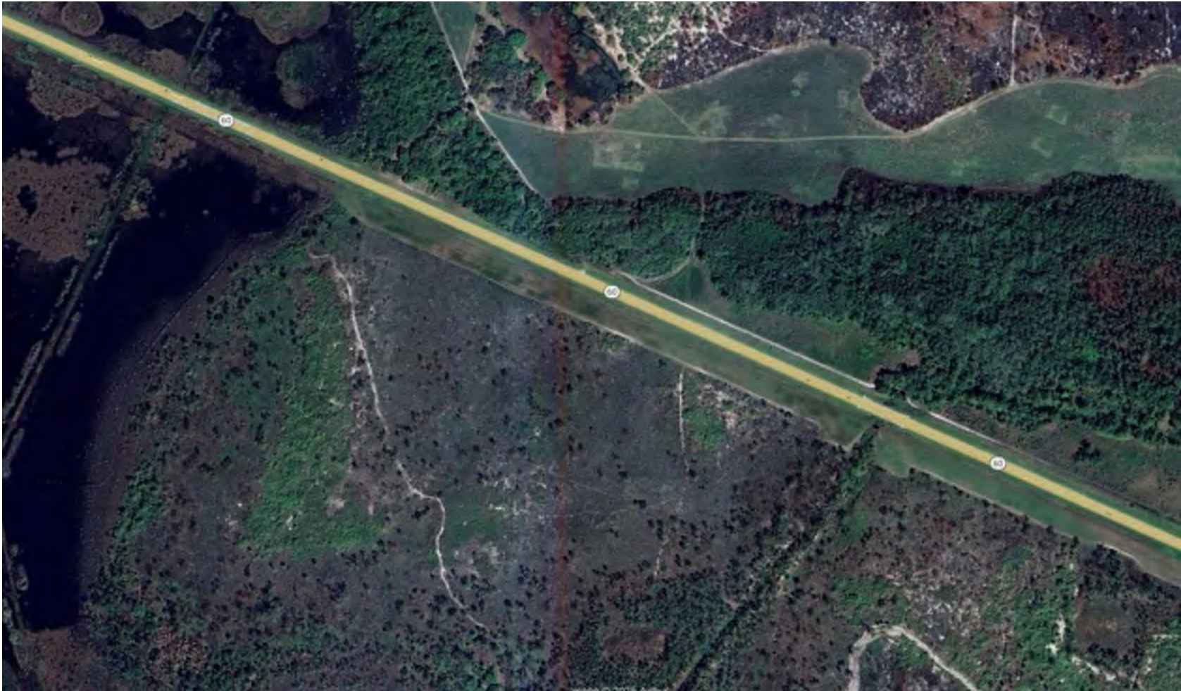
CROWN CASTLE OWNED CONDUIT VIEW
