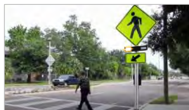
Rectangular Rapid Flashing Beacon
