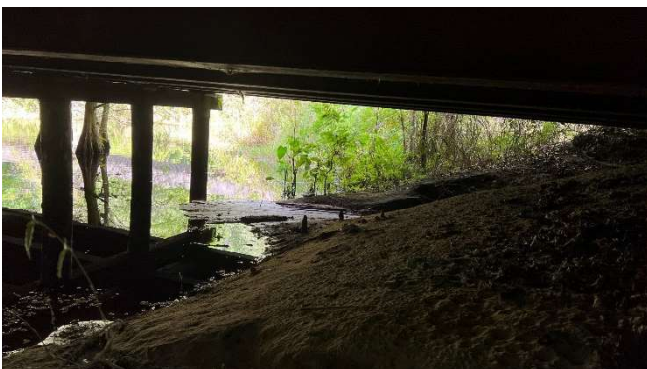
Abutment embankment washout/erosion
