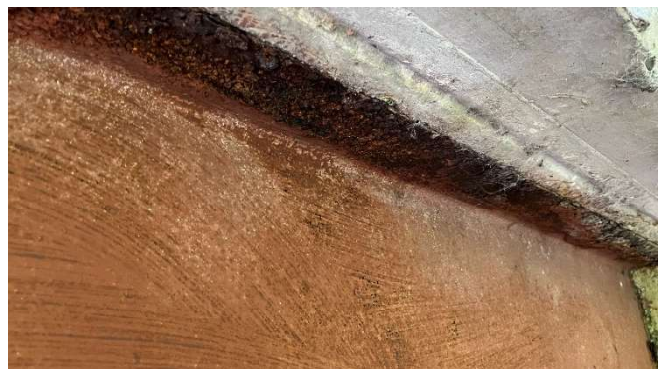
Typical top flange heavy rusting/corrosion
