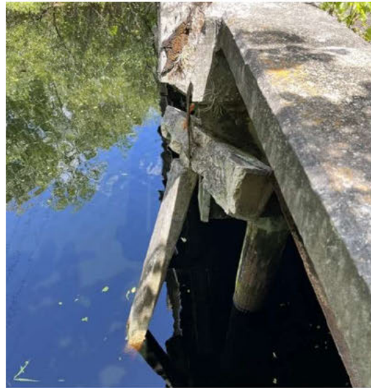
Missing Railing on Historic US 17/92 Bridge
