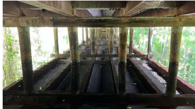
Typical underside view with bent cap repairs
