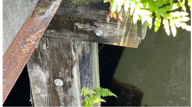
Timber bent cap and pile deterioration and repairs
