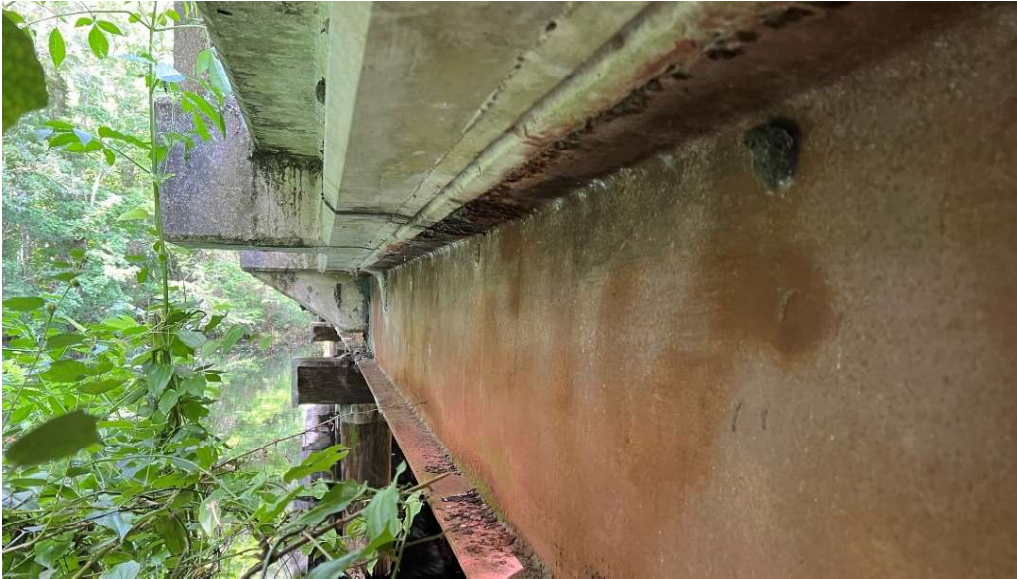
Exterior girder showing signs of heavy corrosion/rusting along the outside flanges. All steel girders show signs of poor maintenance and would, at a minimum, need cleaning and painting.
