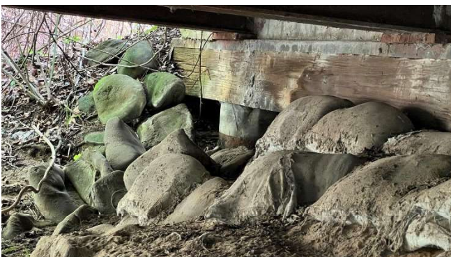
Attempted/failed mitigation of abutment washout
