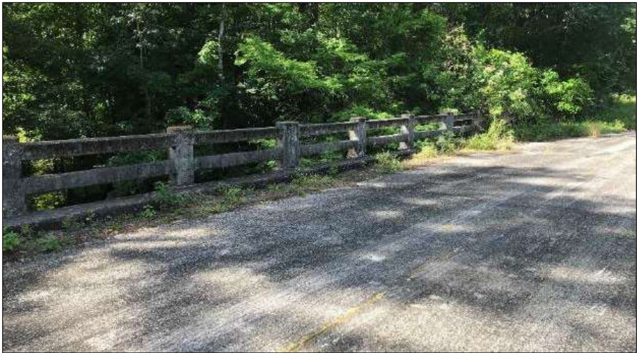
Figure 9. Typical bridge railing that does not meet the Manual for Assessing Safety Hardware (MASH) criteria. Constructing a similar railing to match the design of this historic railing and also meet MASH criteria is not possible. Source: VHB 2022.
