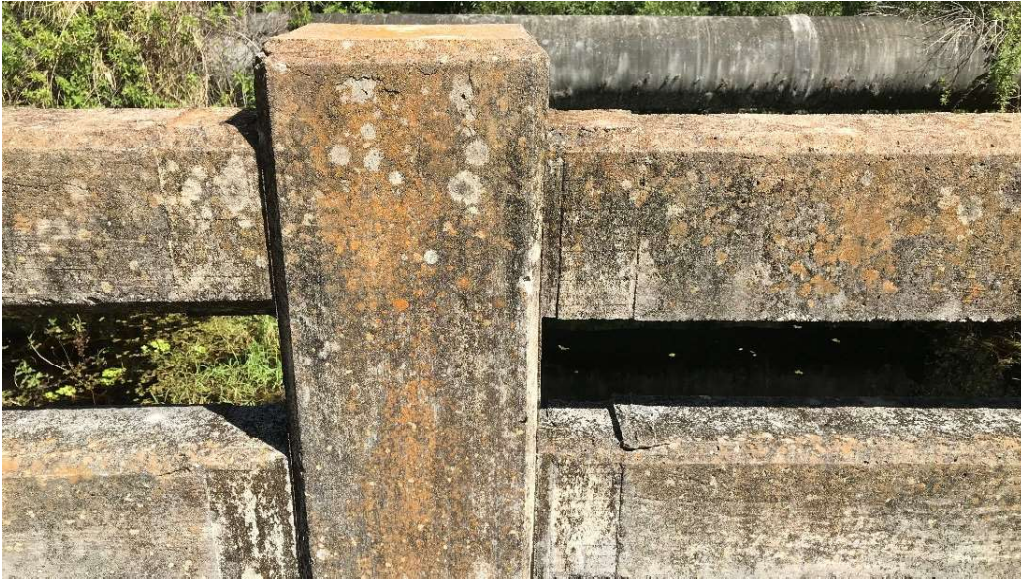
Typical concrete bridge rail post showing typical deterioration and configuration. Replicating a similar railing meeting currently functional and design requirements would not be feasible.
