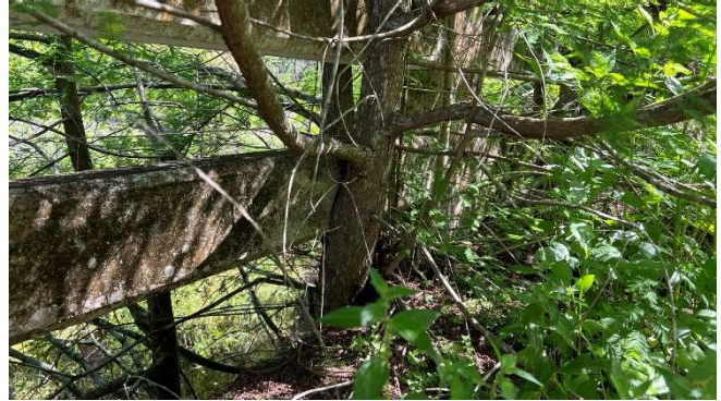
Tree growth through bridge railing and deck
