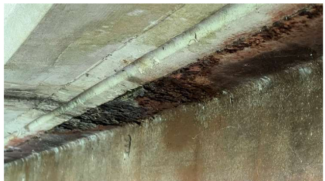
Typical top flange heavy rusting/corrosion
