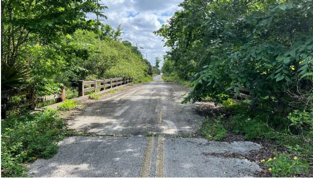
Bridge approach with overgrowth and missing railing
