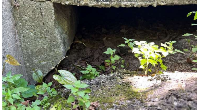
Fully undermined bridge approach and abutment
