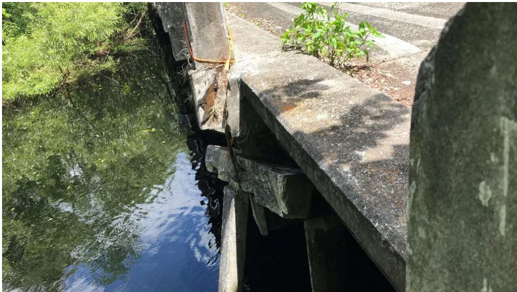
Missing / damaged bridge rail Section showing the apparent lack of reinforcing within the 1930s Bridge Rail System
