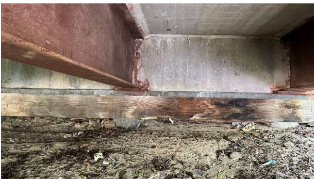
Abutment bent cap with exposed piles/erosion
