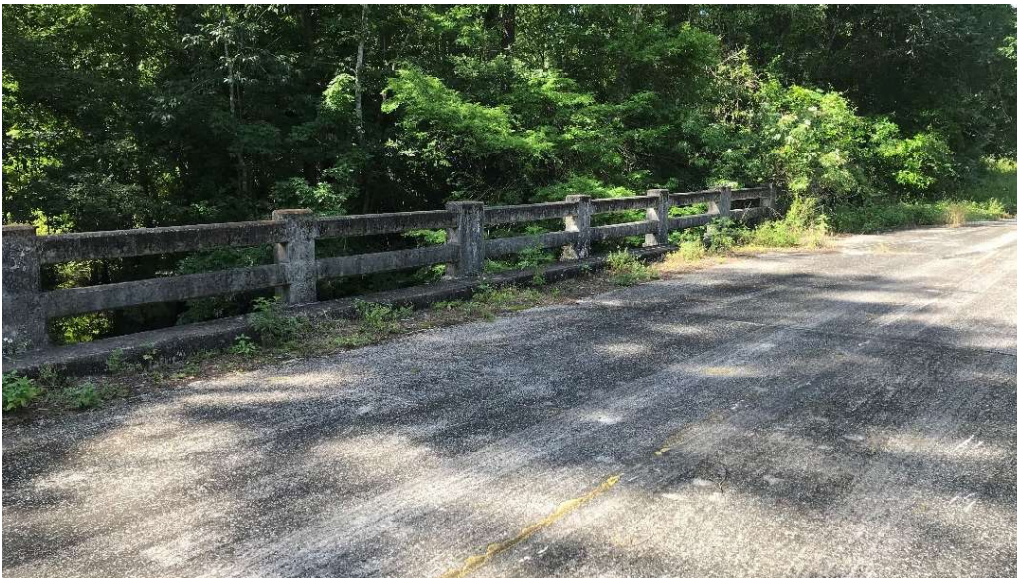
Bridge rail elevation showing the standard 1930s bridge rail (Standard Index No. 1332) that doesn't meet today's AASHTO/FHWA Manual for Assessing Safety Hardware (MASH) crash criteria due to a lack of reinforcement.
