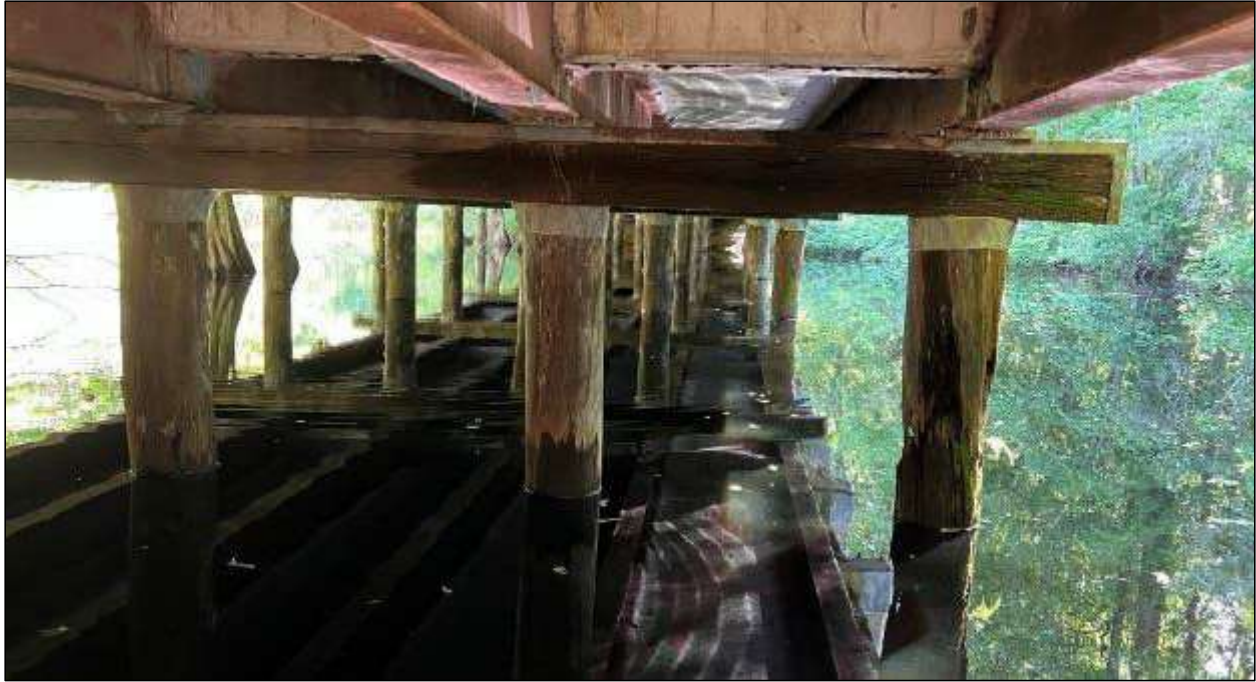
Figure 8. Timber Bents showing decay. Source: VHB 2022.
