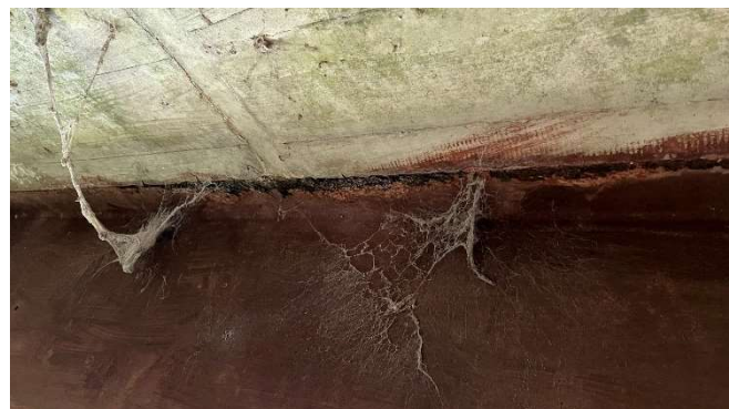
Typical top flange heavy rusting/corrosion
