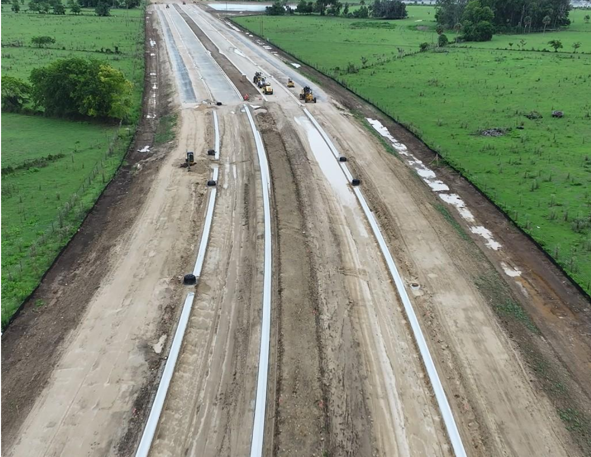
Construction work on new segment of U.S. 301
