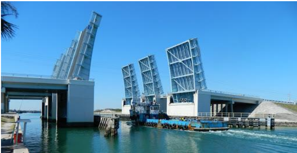
Figure 3: Existing SR 401 Bridges Source: ReelEstateBrevard.com
