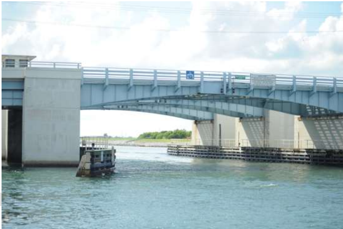
Figure 4-1 Existing S.R. 401 Bascule Bridges (No Build Alternative)
