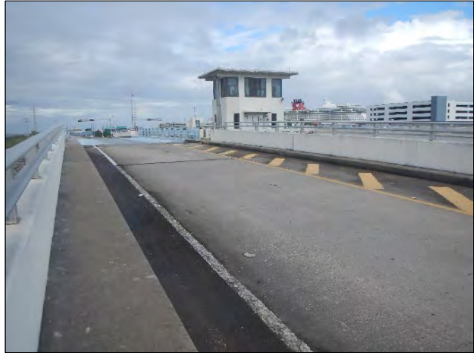
Figure 15. Resource 8BR03010, facing northeast.
