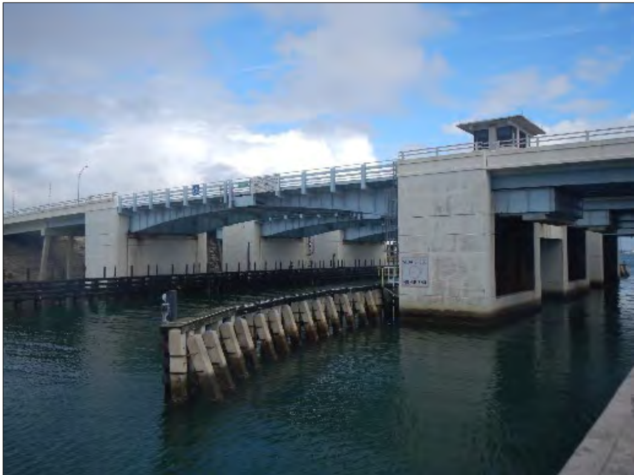
Figure 16. Resource 8BR03010, facing northeast.
