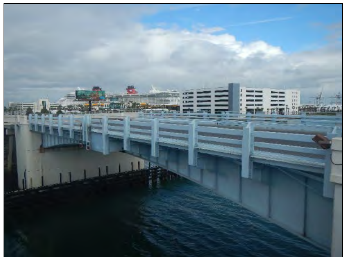
Figure 17. Resource 8BR03395, facing northeast.
