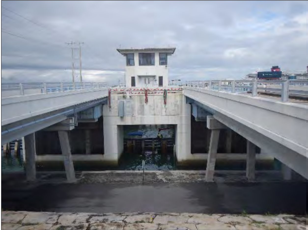
Figure 13. Resource 8BR03010, left. Tender station, center. Resource 8BR03009, right, facing north.
