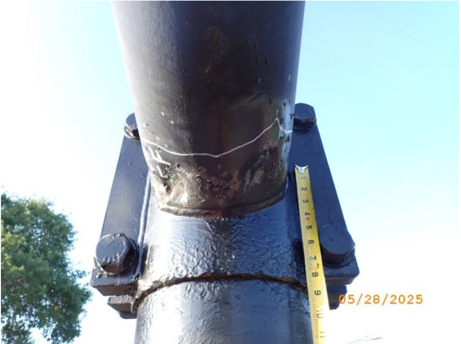
Photo 17 - Element 8484 / Metal Mast Arm Horizontal
