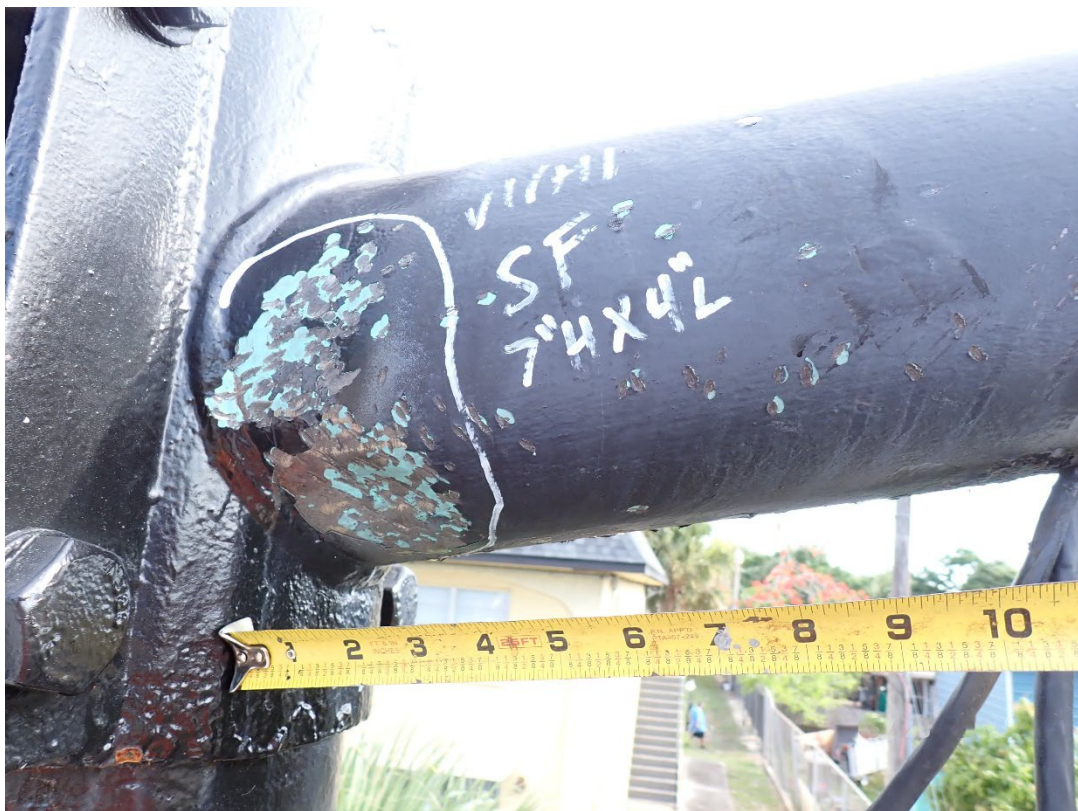
Photo 6: V1/H1 – Slightly malleable area on south face of arm
