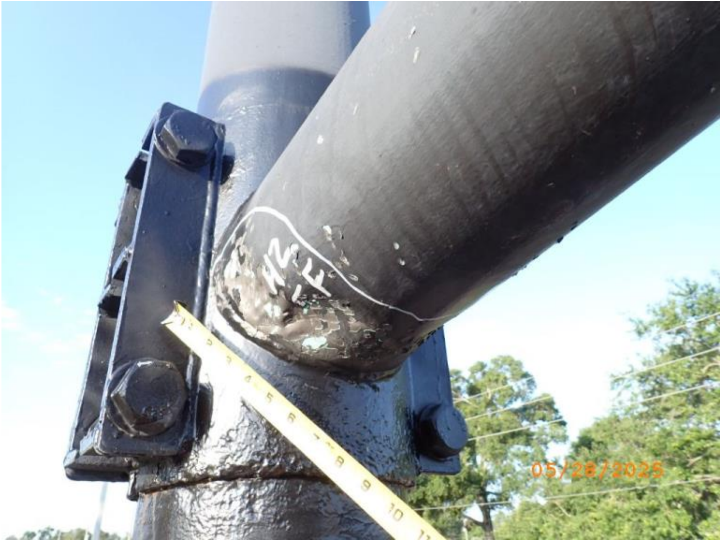
Photo 16 - Element 8484 / Metal Mast Arm Horizontal
