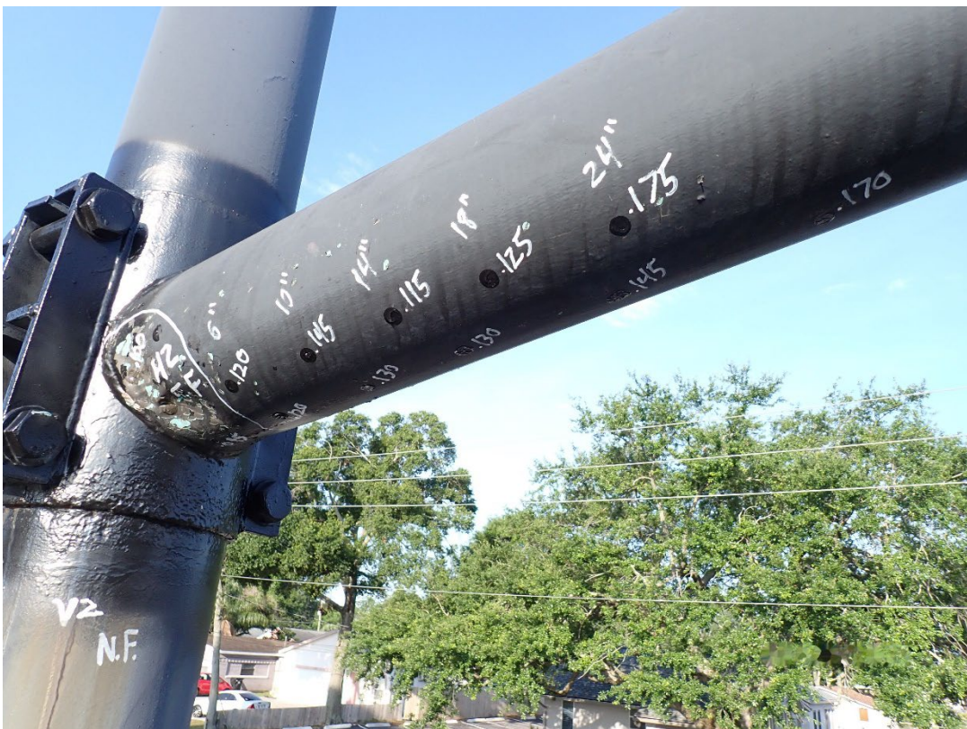
Photo 4: V2/H2 – Thickness readings on underside and east face of arm
