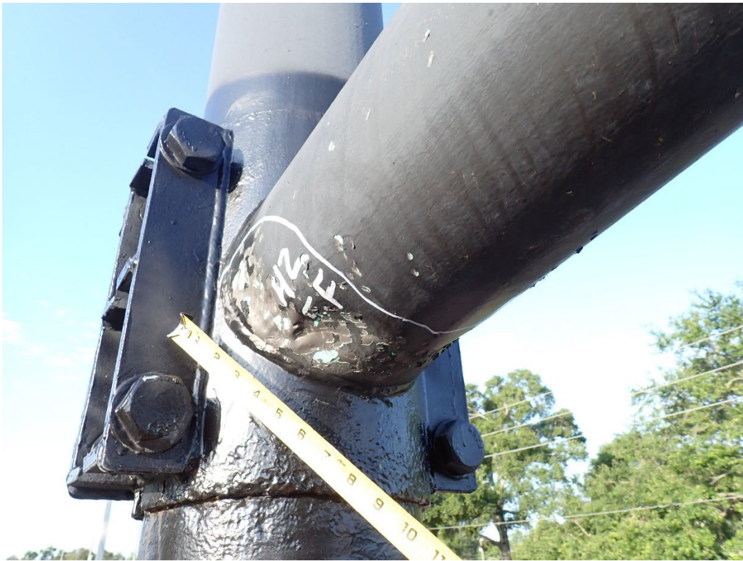
Photo 1: V2/H2 – Malleable area on underside of arm
