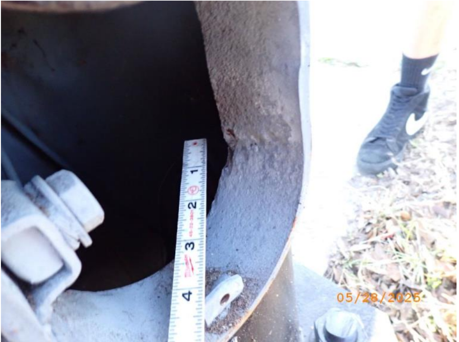
Photo 10 - Element 8481 / Metal Mast Arm Vertical
