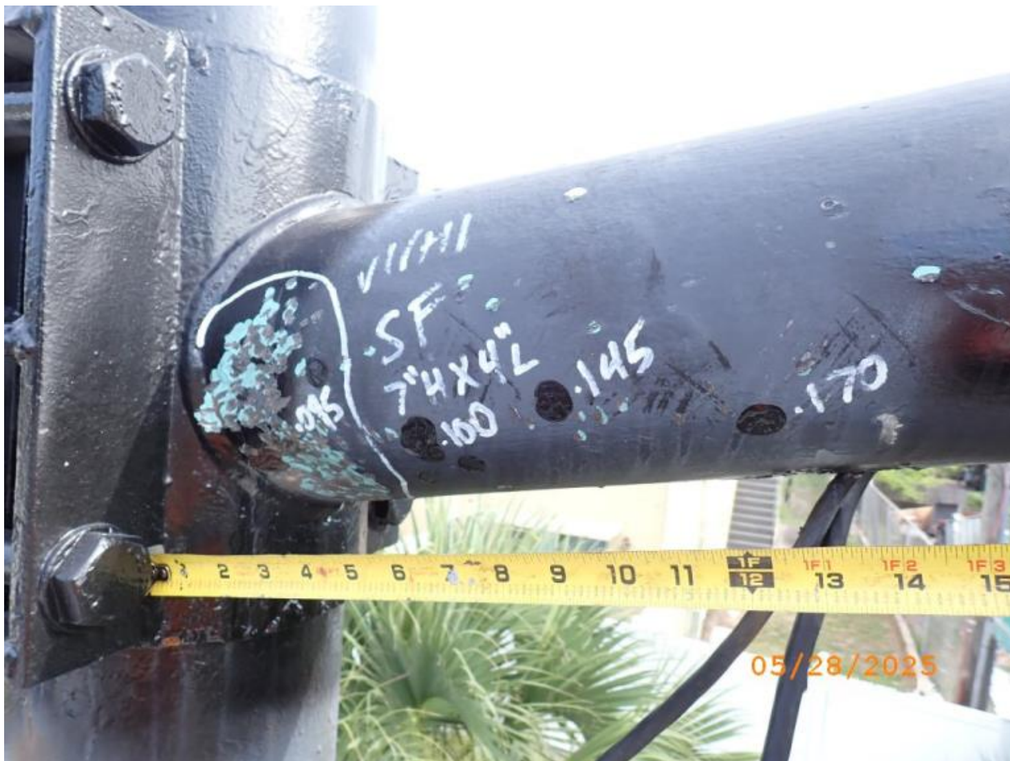
Photo 11 - Element 8484 / Metal Mast Arm Horizontal
