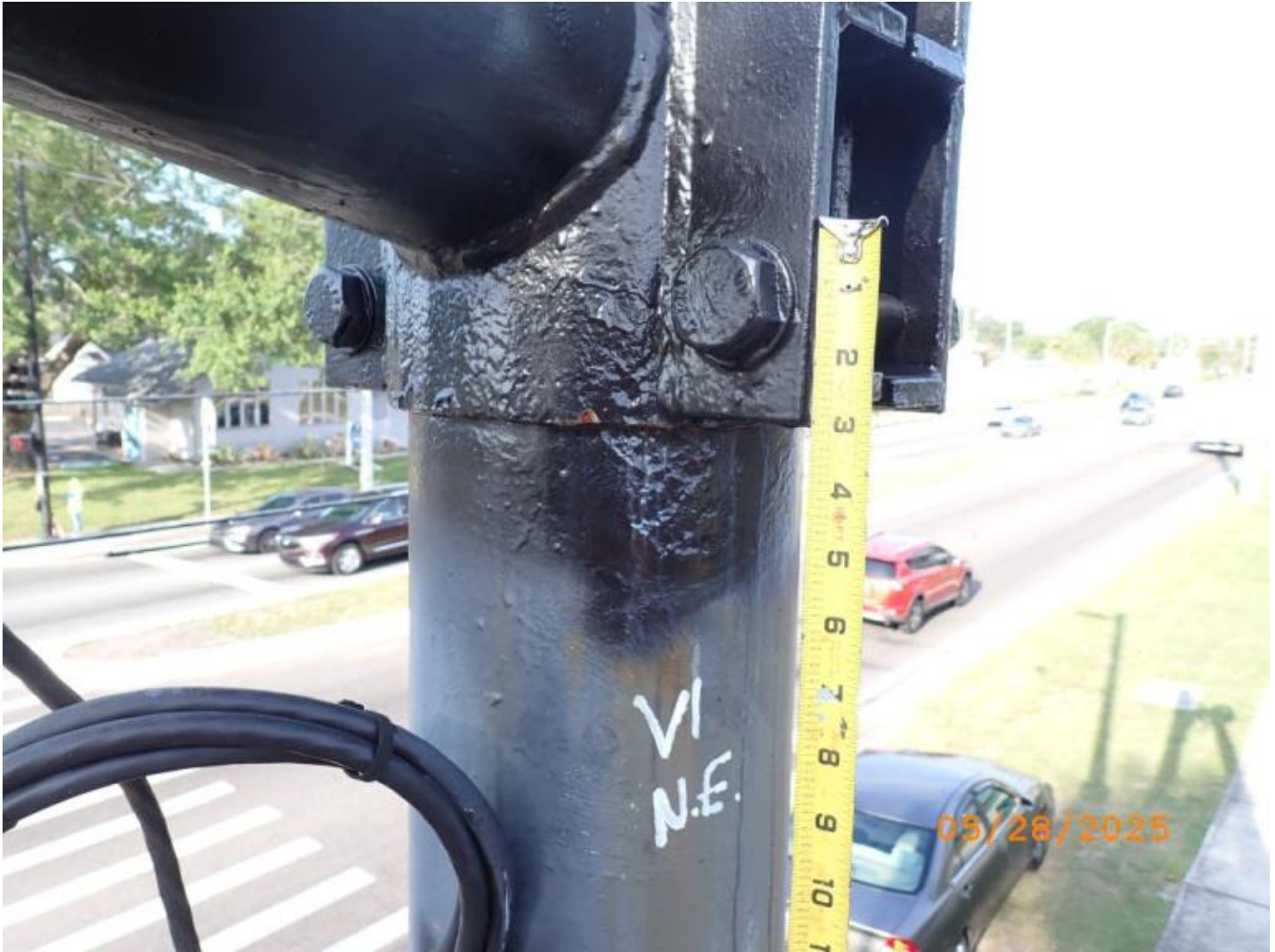
Photo 5 - Element 8481 / Metal Mast Arm Vertical
