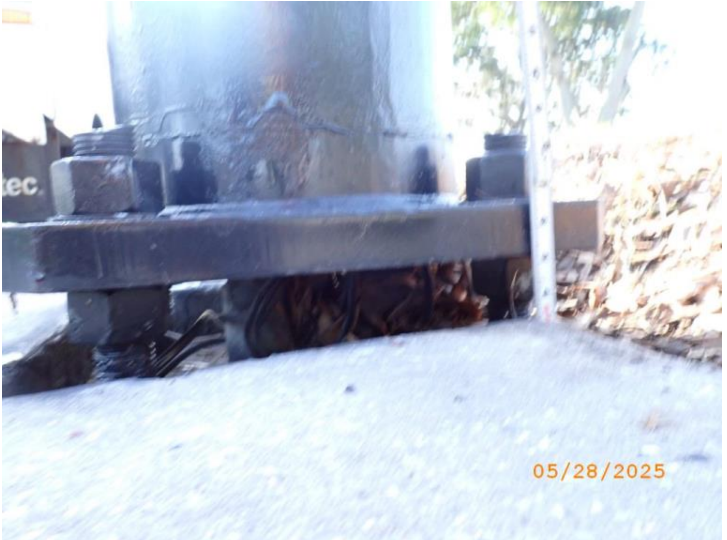
Photo 2 - Element 8480 / Mast Arm Foundation
