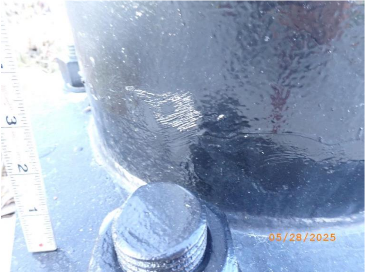
Photo 6 - Element 8481 / Metal Mast Arm Vertical
