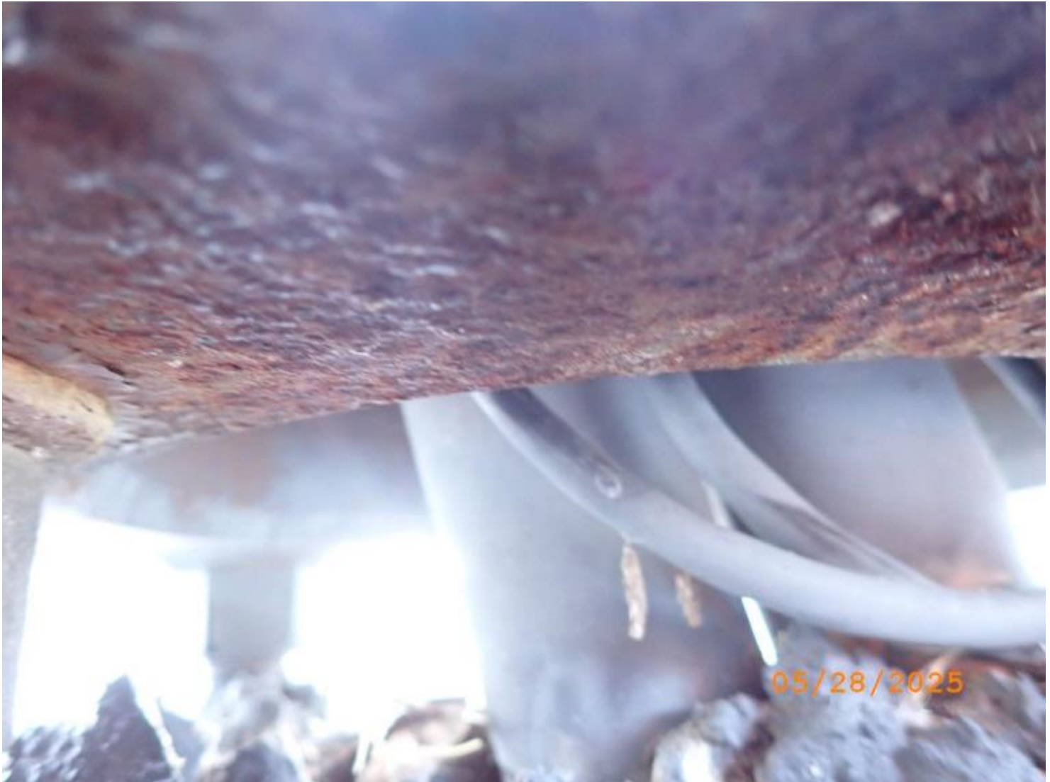
Photo 3 - Element 8481 / Metal Mast Arm Vertical
