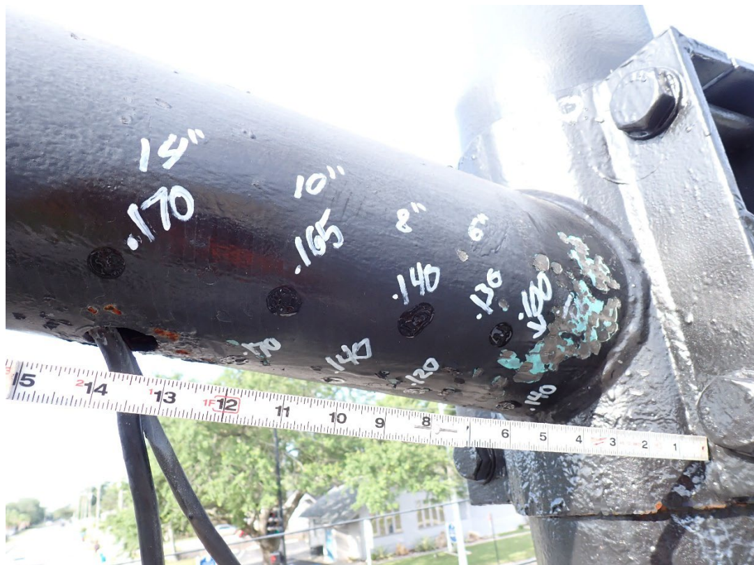
Photo 8: V1/H1 – Thickness readings on underside and north face of arm
