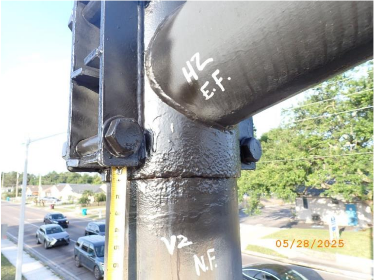
Photo 7 - Element 8481 / Metal Mast Arm Vertical
