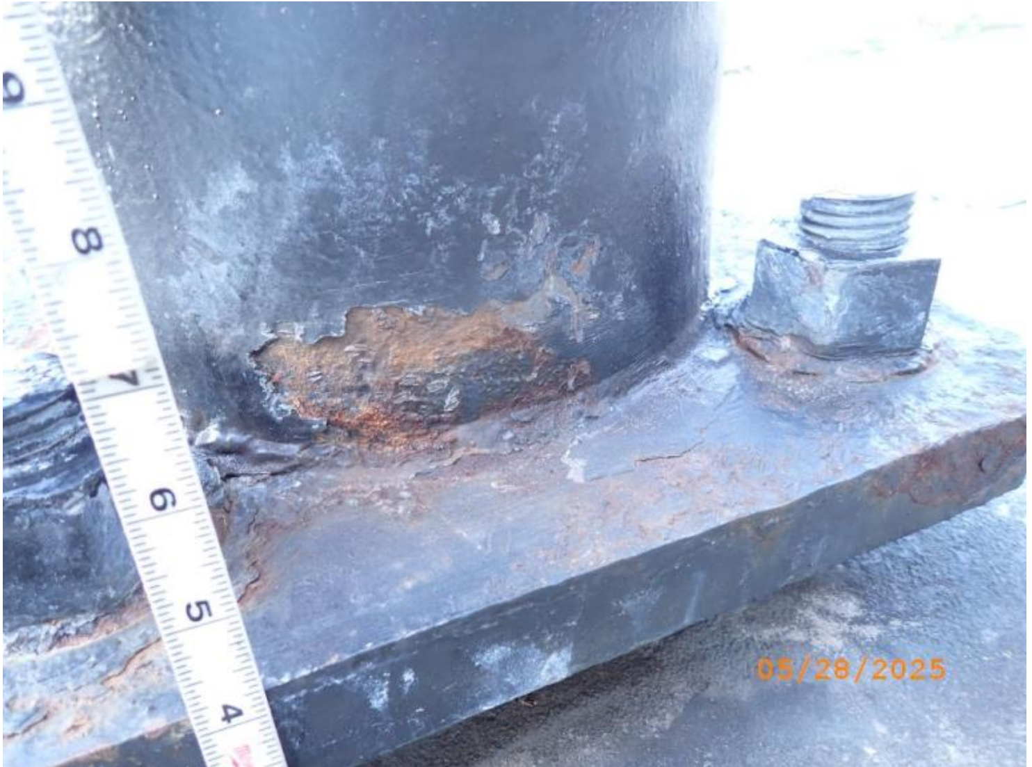
Photo 4 - Element 8481 / Metal Mast Arm Vertical
