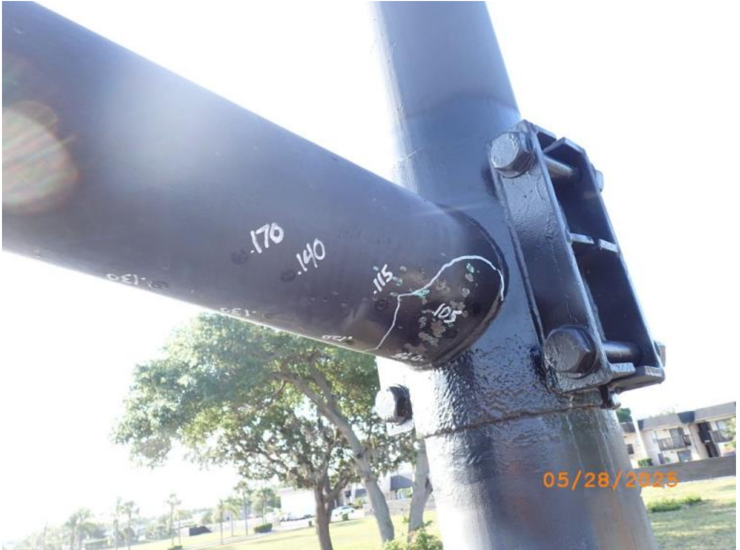
Photo 20 - Element 8484 / Metal Mast Arm Horizontal
