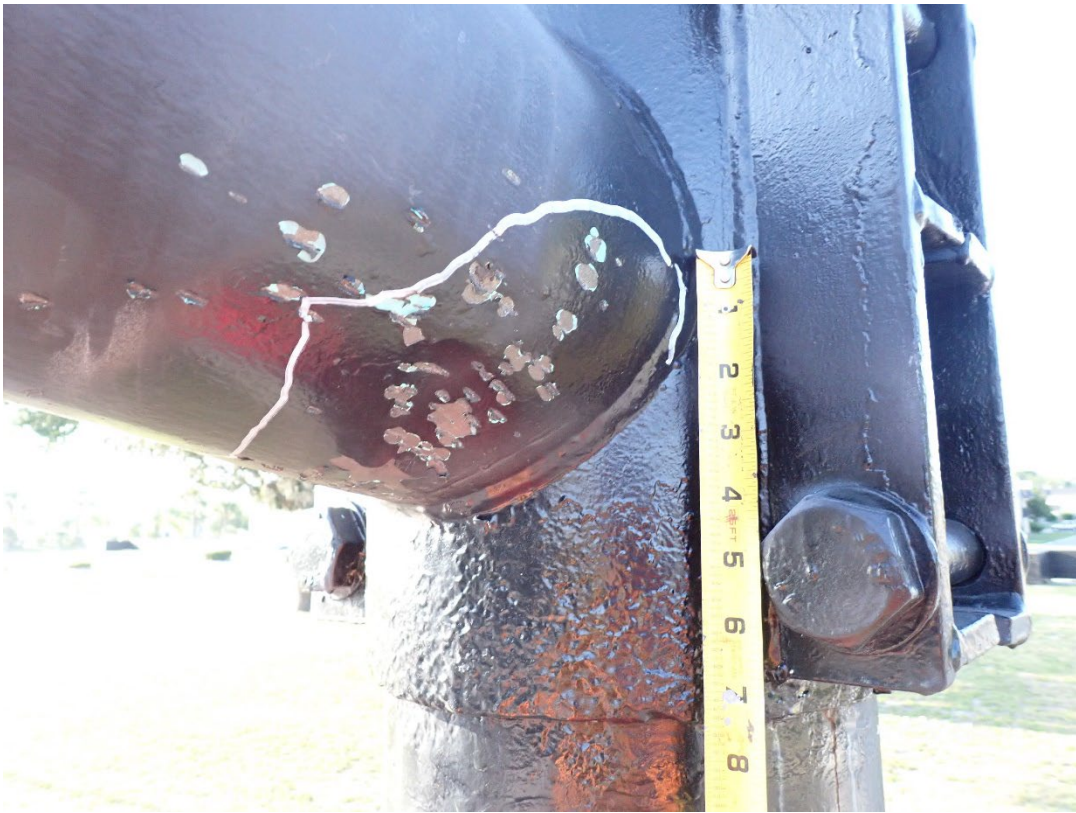
Photo 3: V2/H2 – Malleable area on underside of arm
