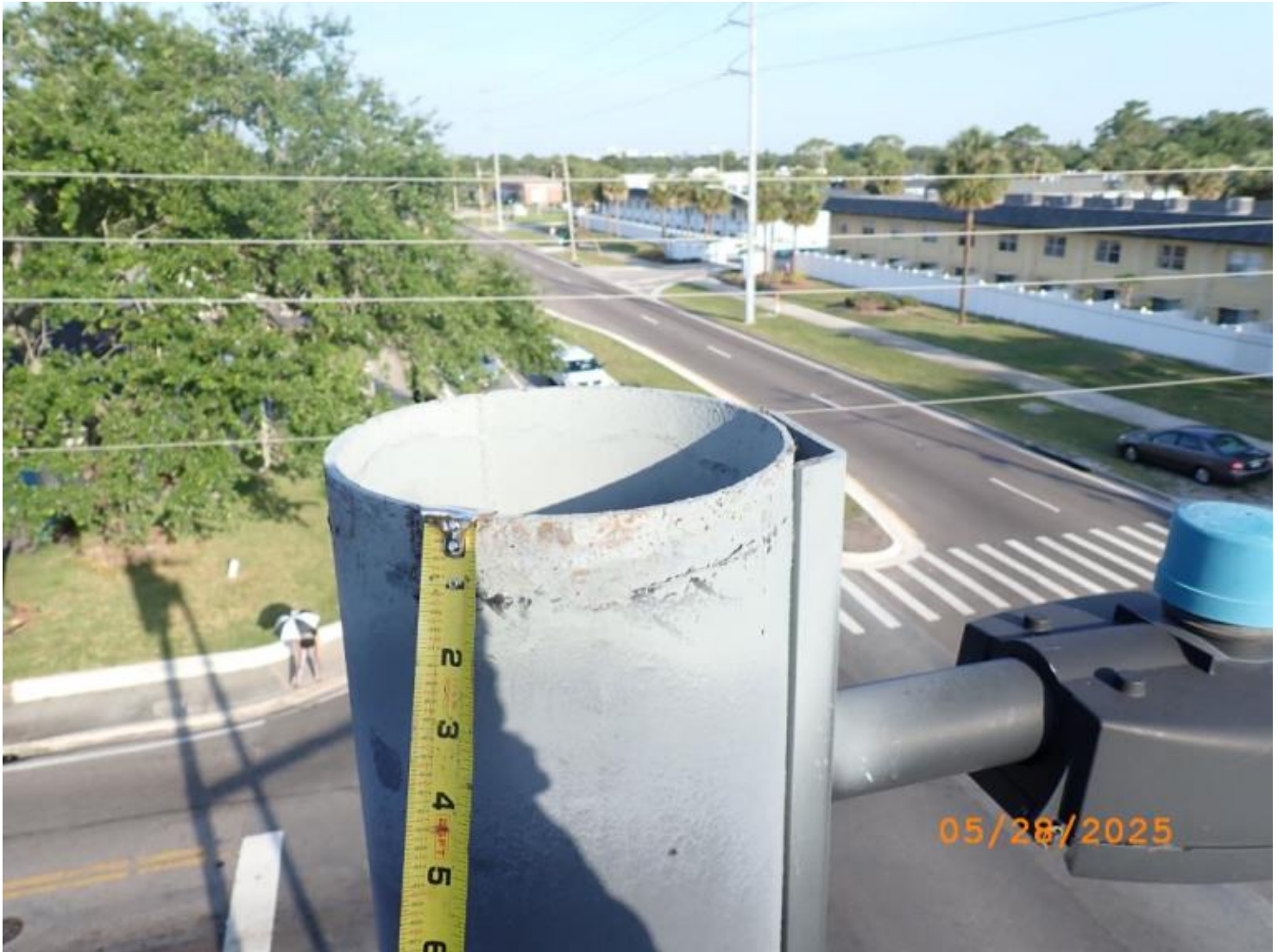
Photo 9 - Element 8481 / Metal Mast Arm Vertical
