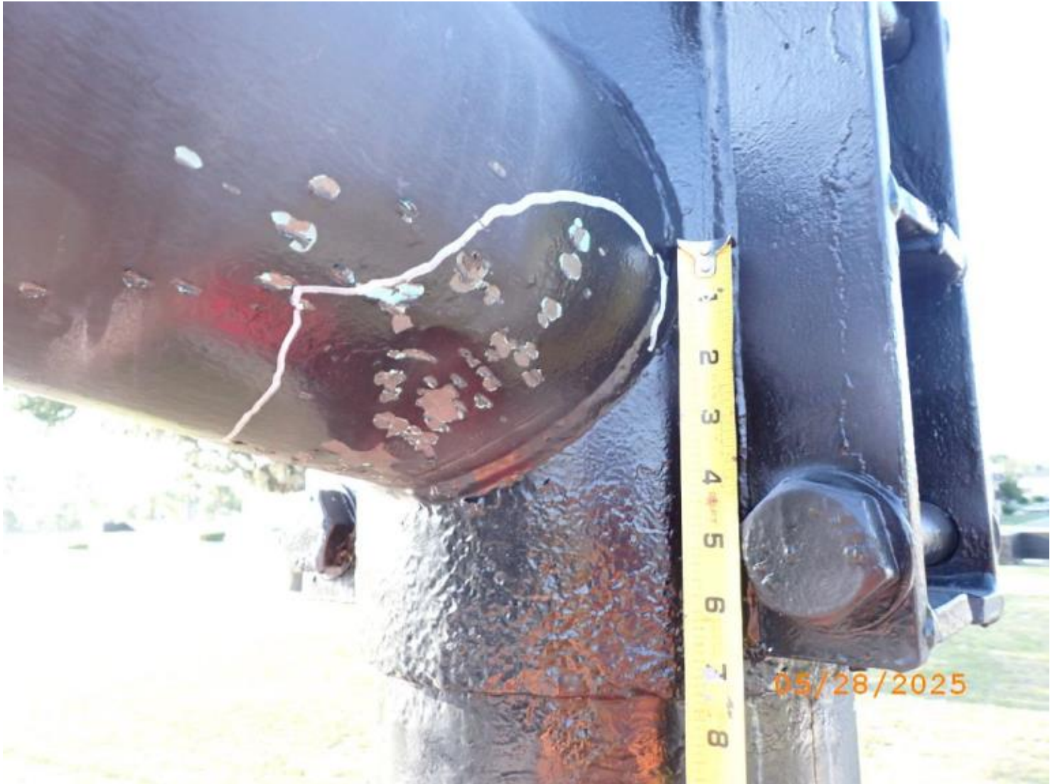
Photo 18 - Element 8484 / Metal Mast Arm Horizontal
