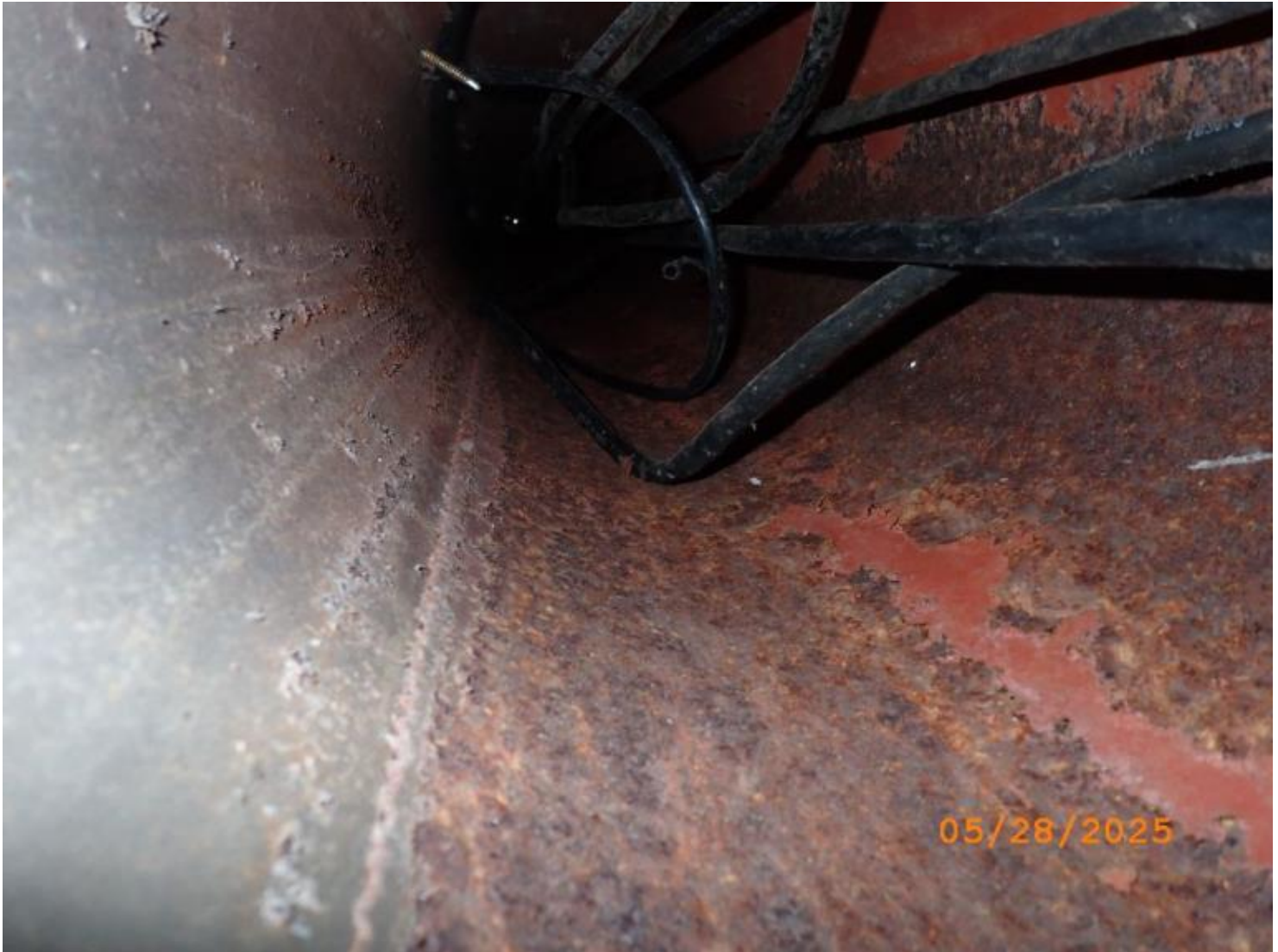
Photo 8 - Element 8481 / Metal Mast Arm Vertical
