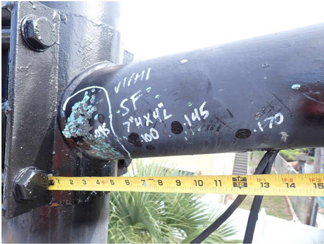
Photo 7: V1/H1 – Thickness readings on south face of arm
