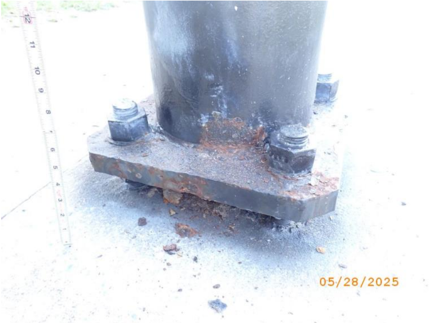
Photo 1 - Element 8480 / Mast Arm Foundation
