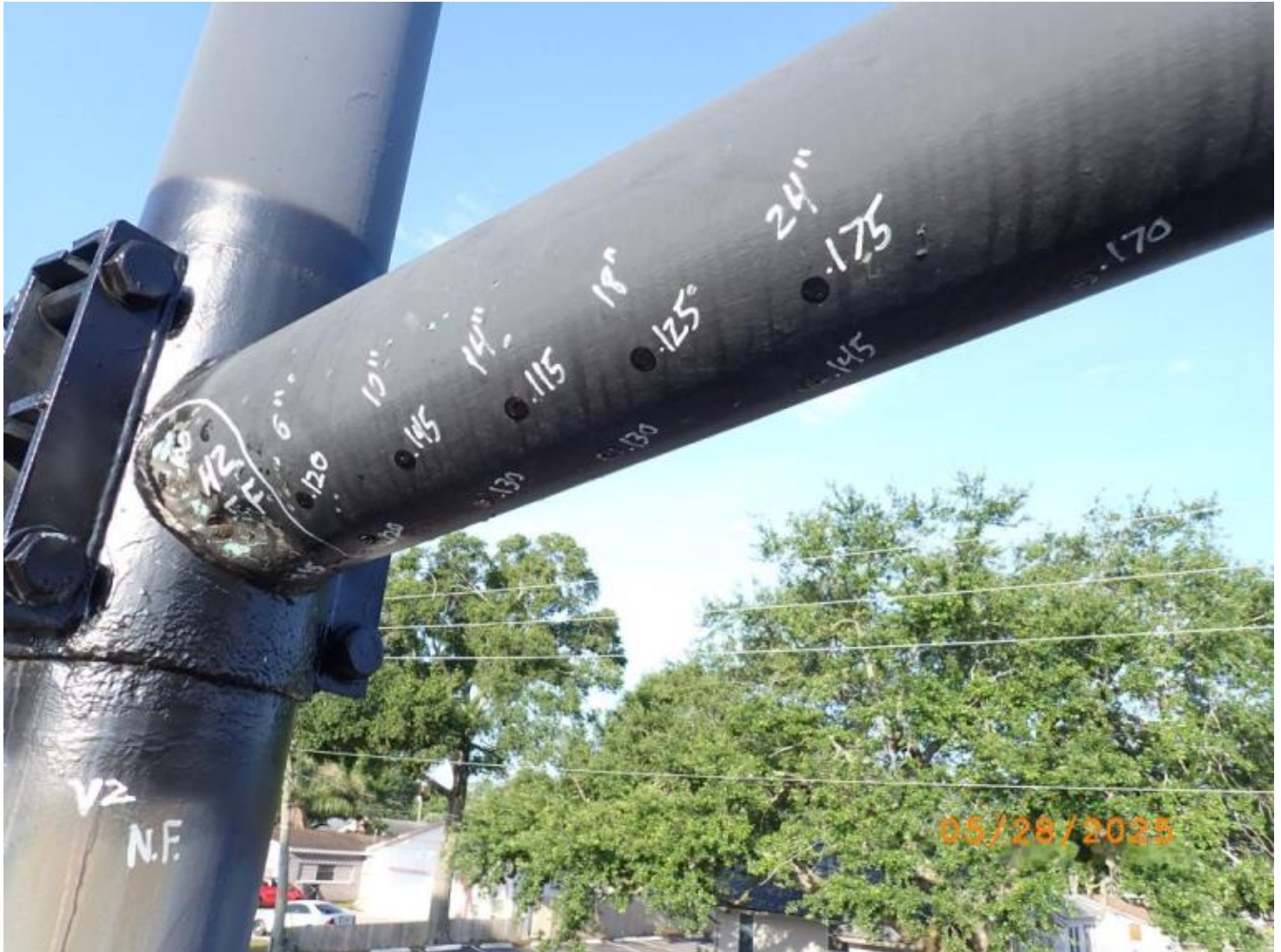
Photo 19 - Element 8484 / Metal Mast Arm Horizontal
