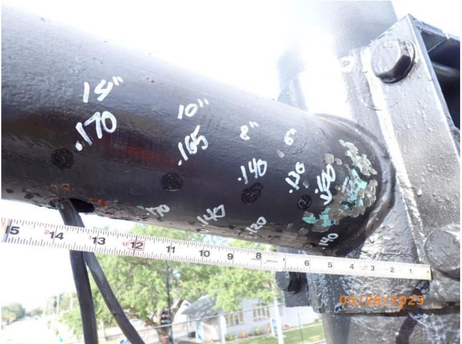
Photo 12 - Element 8484 / Metal Mast Arm Horizontal
