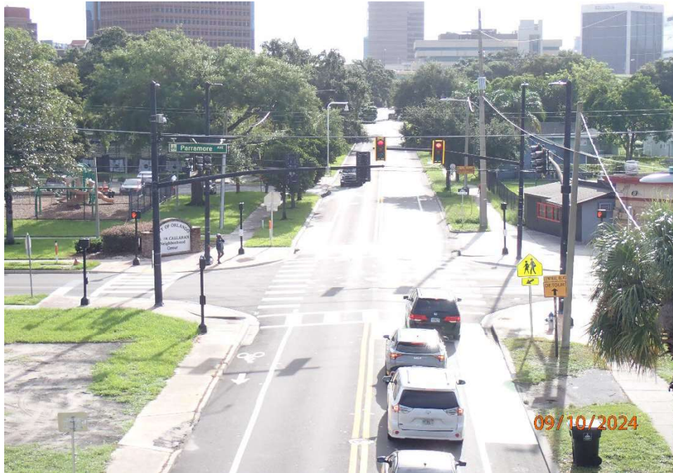
Structure Inventory Photo
