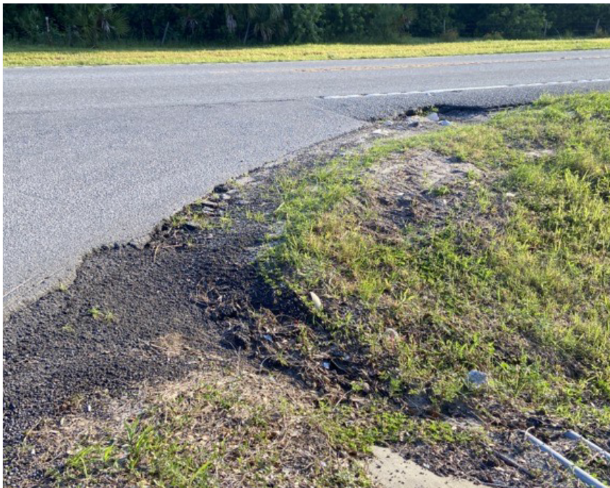
Figure 4-9 Edge Failure on Richmond Avenue East Edge of Pavement
