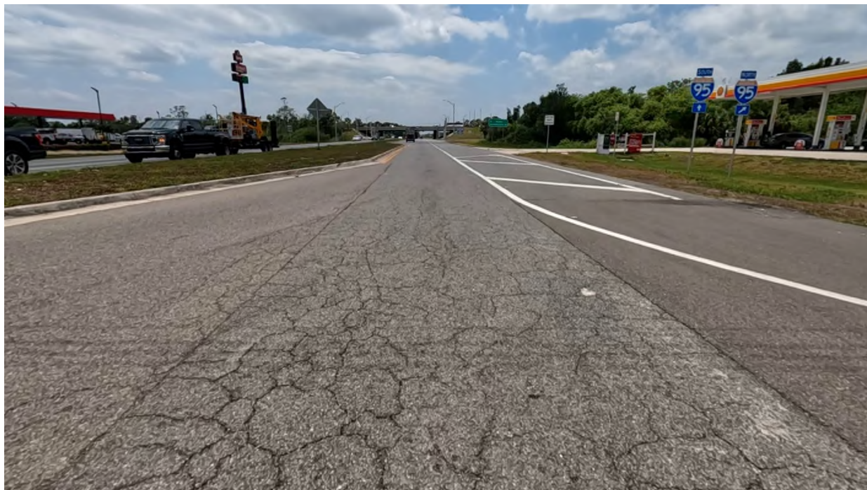
Photo 10: SR 524 Southbound, L1 near MP 1.836, alligator cracking and joint separation at the intersection of SR 524 and Friday Rd.
