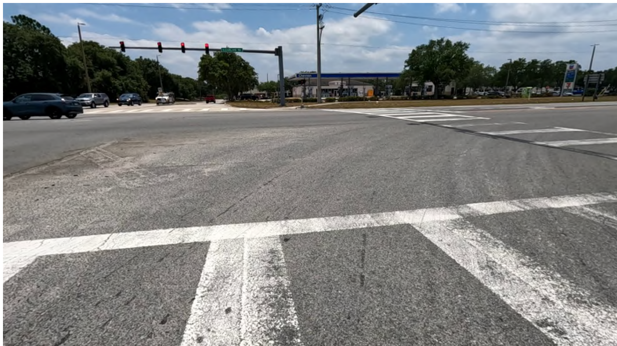
Photo 6: SR 524 Southbound, L1 near MP 5.212, wearing of friction course with delamination at the intersection of SR 524 and Industry Rd.
