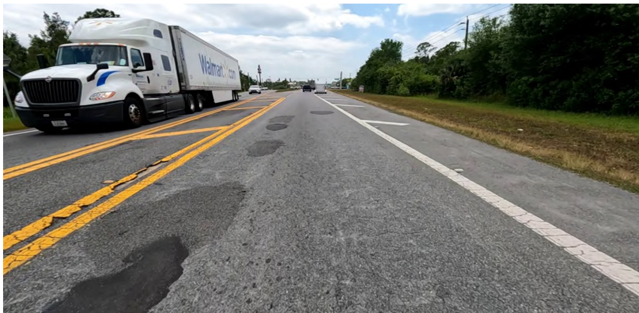
Photo 9: SR 524 Southbound, L1 near MP 1.950, branch cracking with limerock pumping and wearing of friction course with delamination. Note the multiple maintenance/pothole patches.
