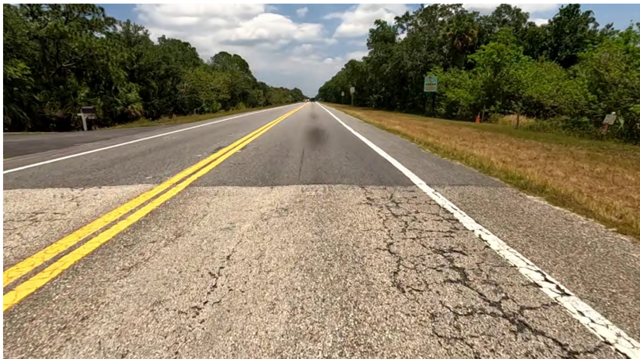
Photo 1: SR 524, Northbound, R1 near MP 0.200, longitudinal and alligator cracking with delamination and pavement change.
