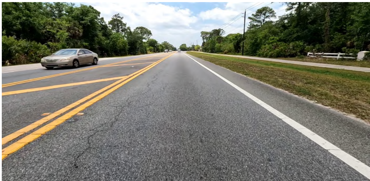
Photo 7: SR 524 Southbound, L1 near MP 2.450, longitudinal and branch cracking.
