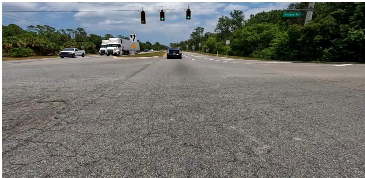
Photo 4: SR 524, Northbound, R1 near MP 1.836, longitudinal and alligator cracking with wearing of friction course and delamination at the intersection of SR 524 and Friday Dr.
