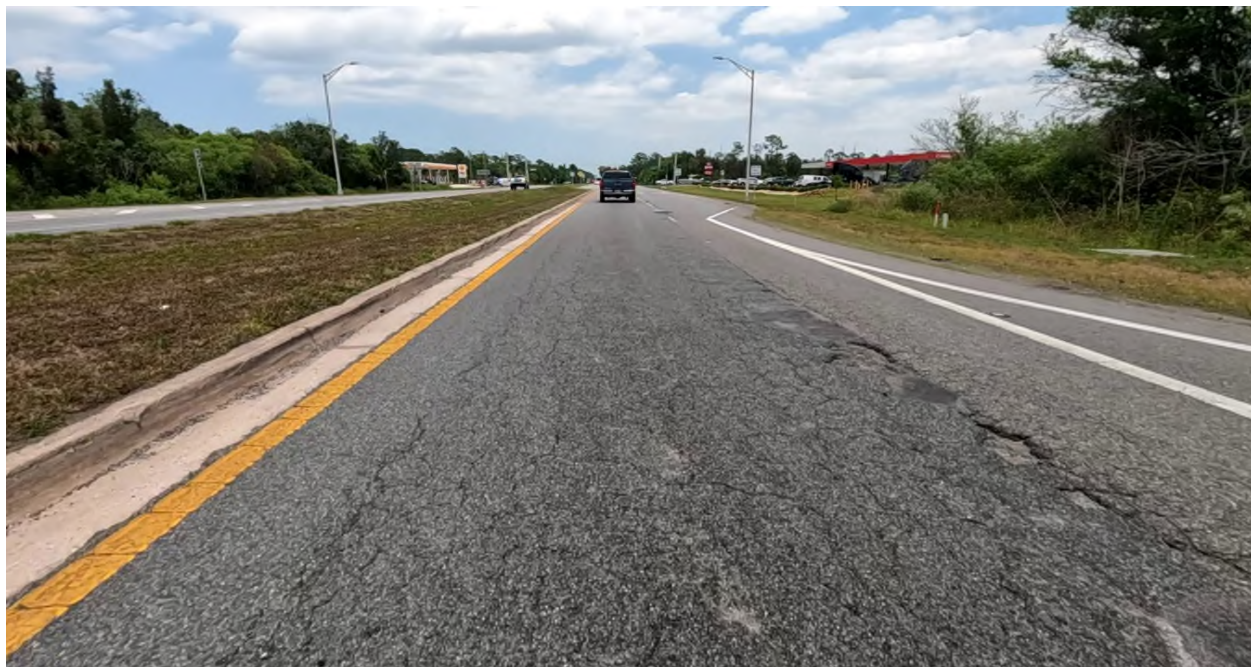
Photo 3: SR 524, Northbound, R1 near MP 1.715, longitudinal and alligator cracking with delamination at I-95 NB Off Ramp.
