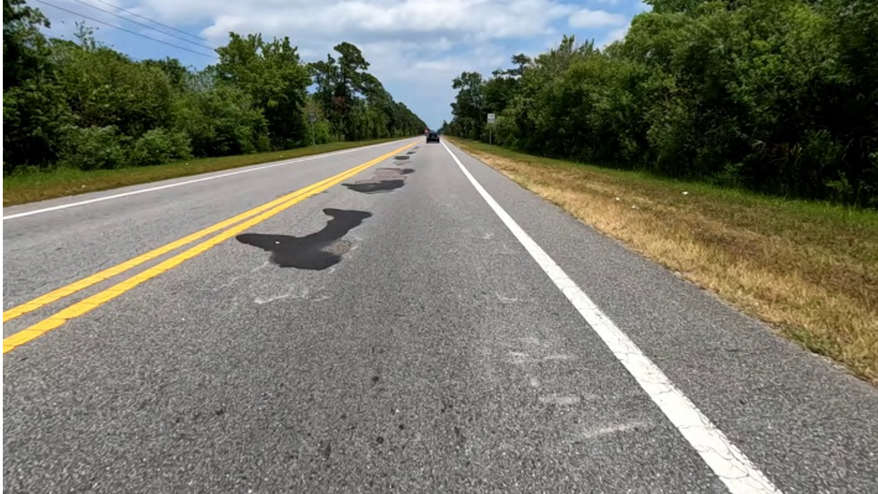
Photo 5: SR 524, Northbound, R1 near MP 1.850, maintenance patches. Note the light branch cracking with limerock pumping.
