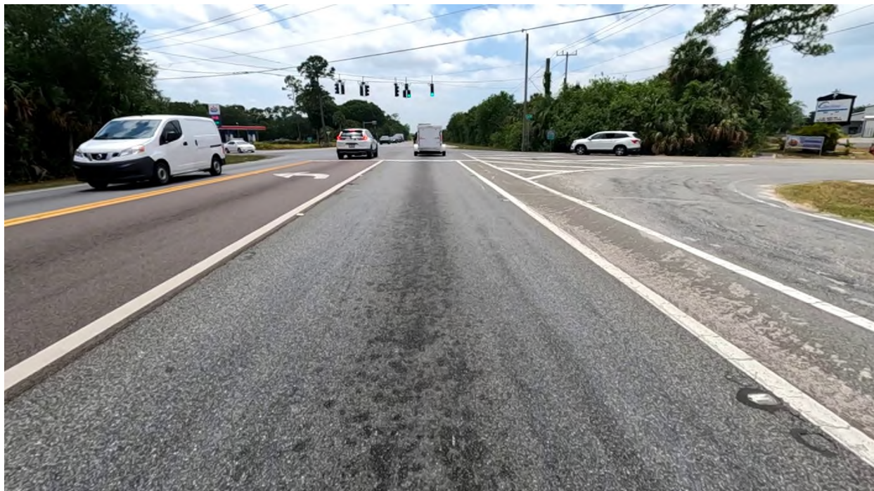
Photo 8: SR 524 Southbound, L1 near MP 2.916, wearing of the friction course with delamination on right turn lane (LRTL) onto Cox Rd.
