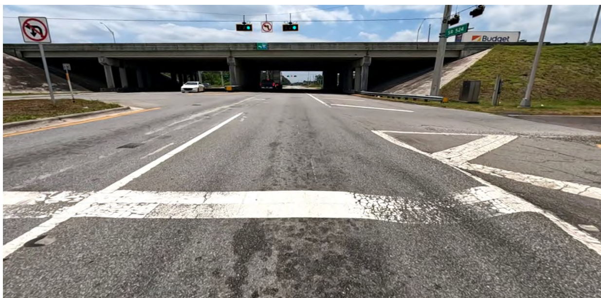
Photo 11: SR 524 Southbound, L1 near MP 1.695, shoving and wearing of friction course at I-95 NB On Ramp. Note the visible rutting in the outside wheelpath.
