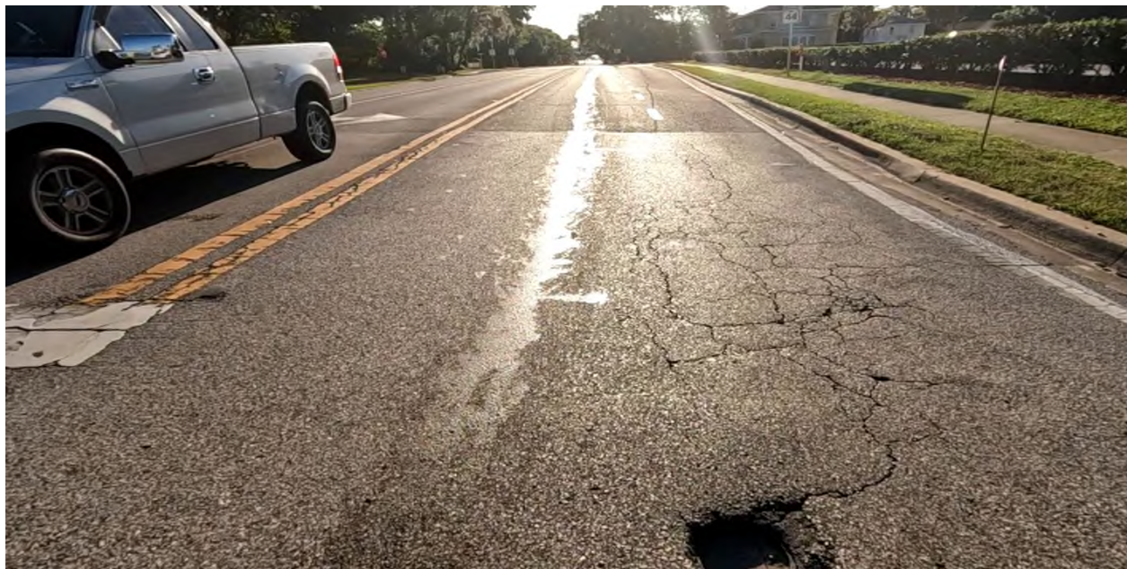
Photo 5: SR 44 Eastbound, R1 near MP 3.867. A view of alligator cracking near utility access cover.
