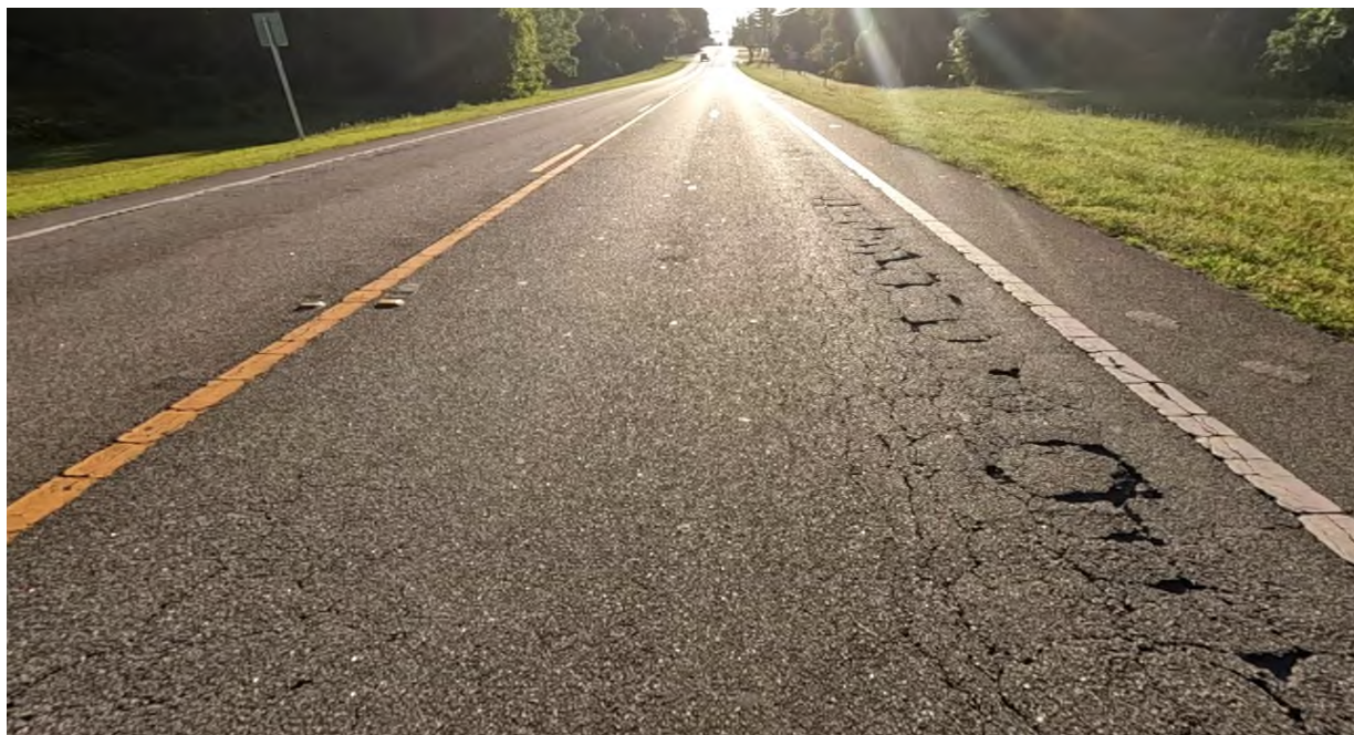
Photo 1: SR 44 Eastbound, R1 near MP 2.856. A view of alligator cracking with asphalt pop-outs.
