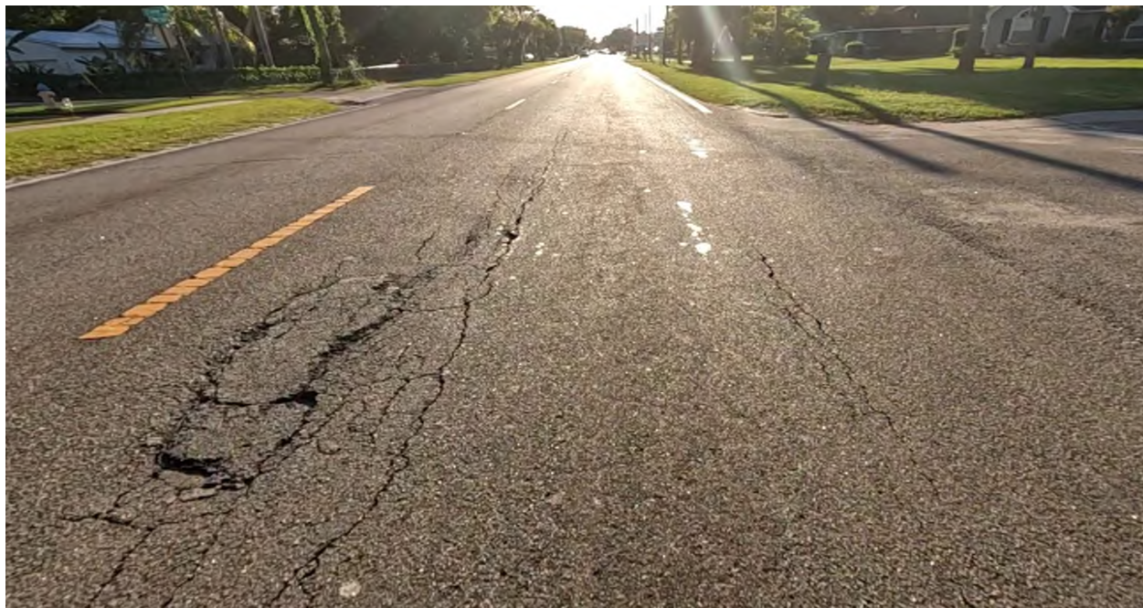
Photo 3: SR 44 Eastbound, R1 near MP 3.708. A view of longitudinal cracking with severe rutting / depression.
