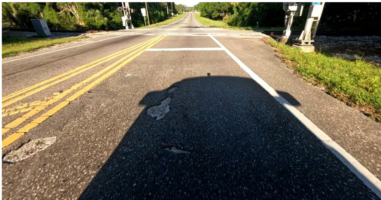
Photo 6: SR 44 Westbound, L1 near MP 3.074. A view of wearing of friction course and delamination near railroad crossing.
