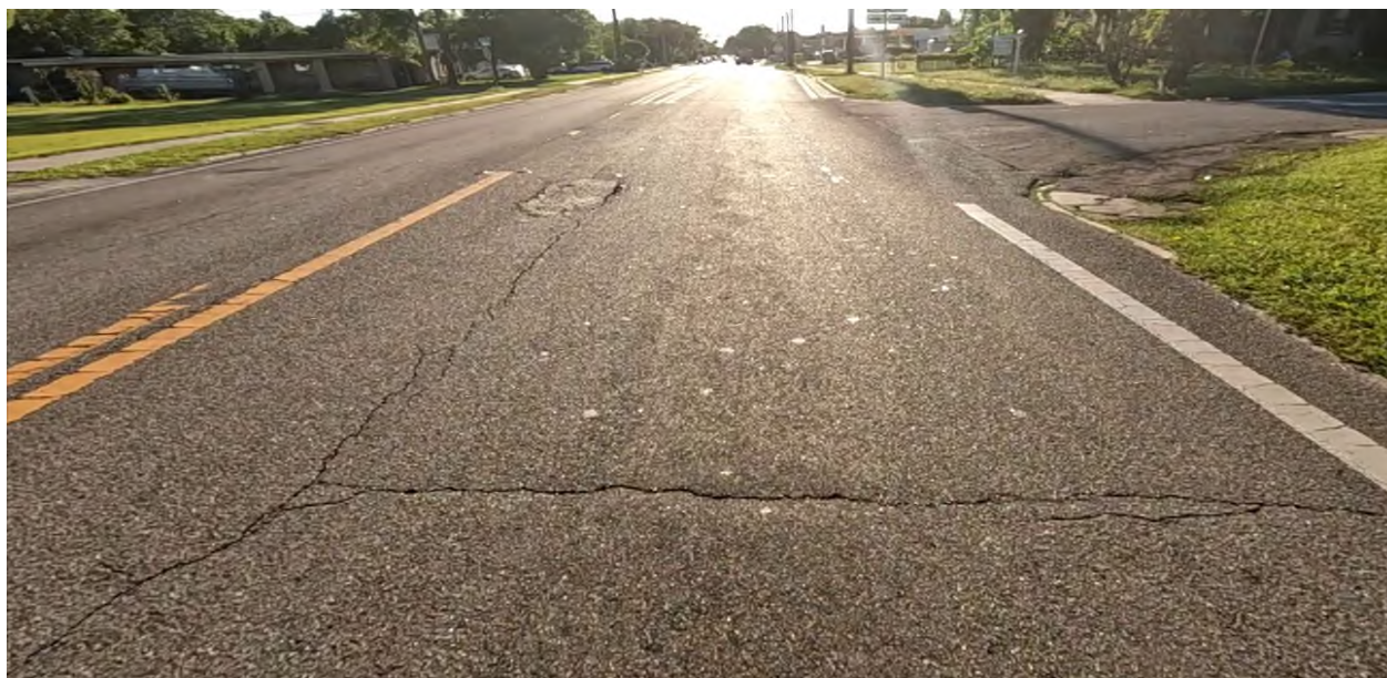
Photo 4: SR 44 Eastbound, R1 near MP 3.773. A view of longitudinal and transverse cracking.
