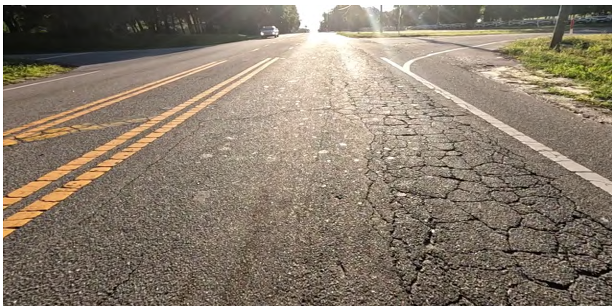
Photo 2: SR 44 Eastbound, R1 near MP 3.108. A view of severe alligator cracking.
