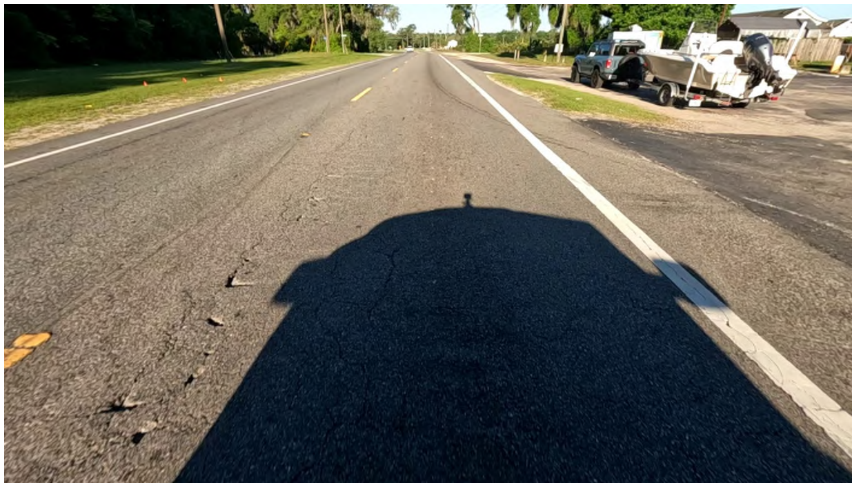
Photo 7: SR 44 Westbound, L1 near MP 2.900. A view of light to moderate branch cracking with asphalt pop-outs.
