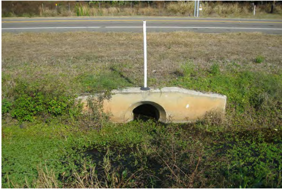
Cross Drain No. 1 – Looking North
