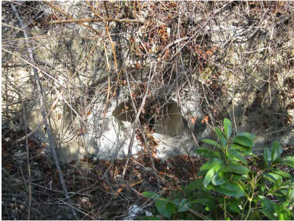
Cross Drain No. 8 – Looking North
