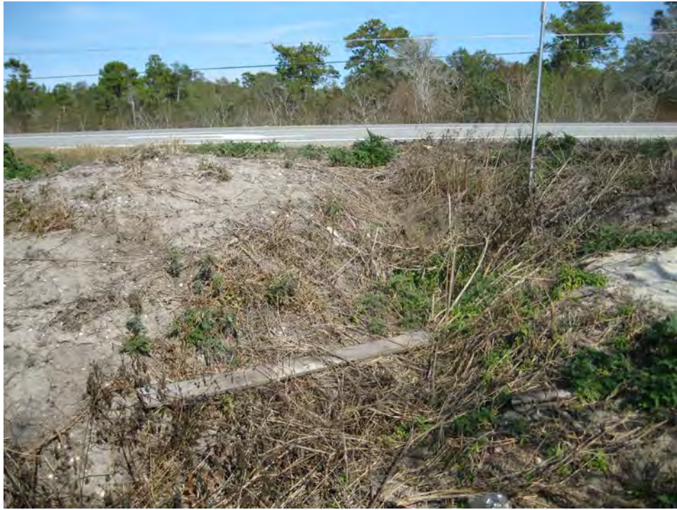
Cross Drain No. 7 – Looking North
