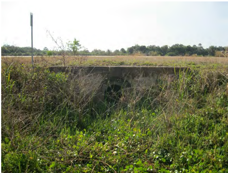
Cross Drain No. 1 – Looking South
