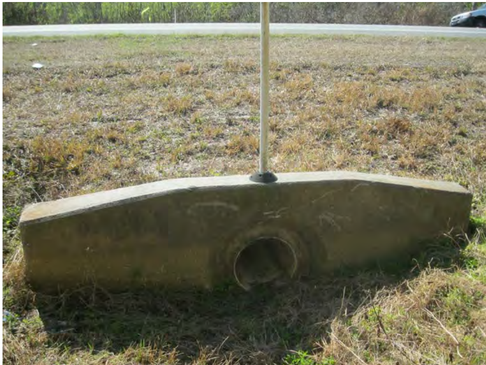
Cross Drain No. 6 – Looking South
