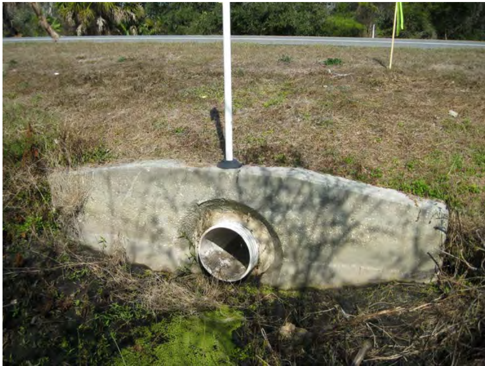
Cross Drain No. 6 – Looking North
