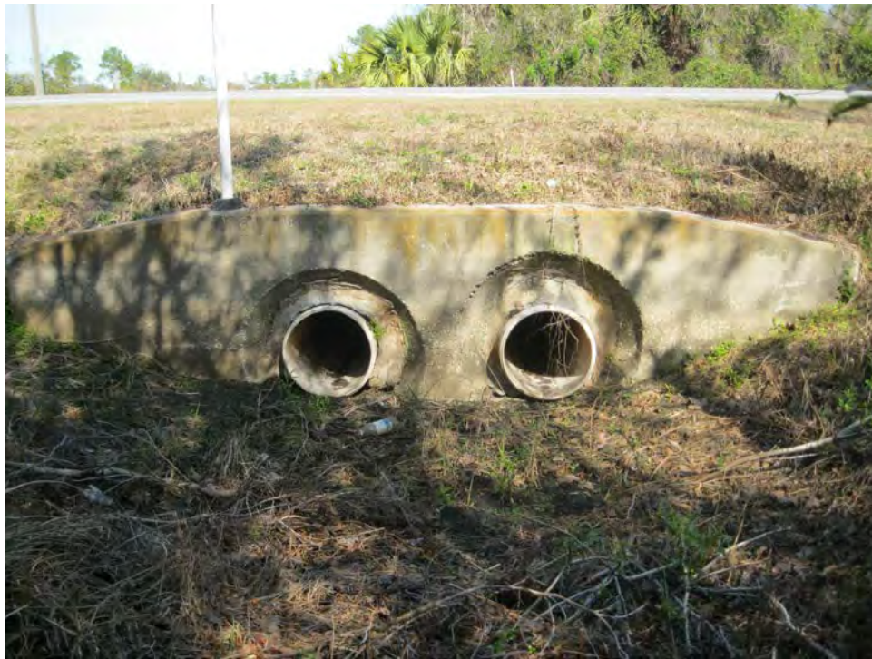
Cross Drain No. 5 – Looking North
