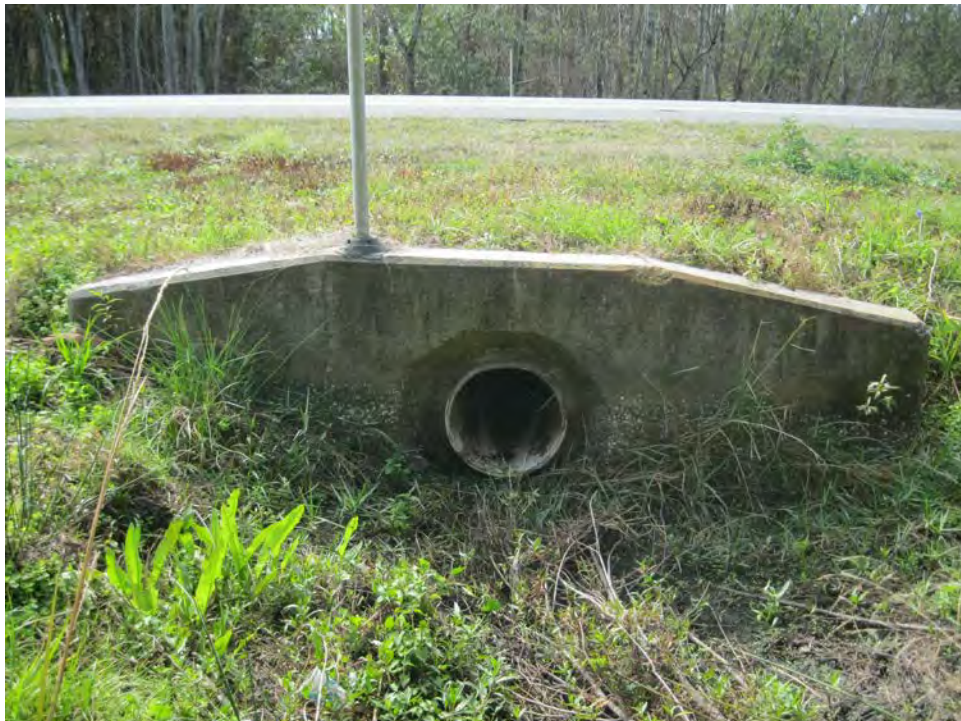
Cross Drain No. 2 – Looking South
