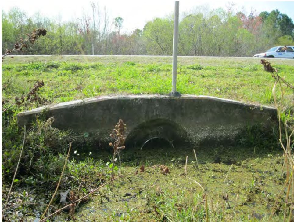
Cross Drain No. 3 – Looking South
