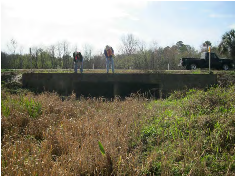
Cross Drain No. 4 – Looking South
