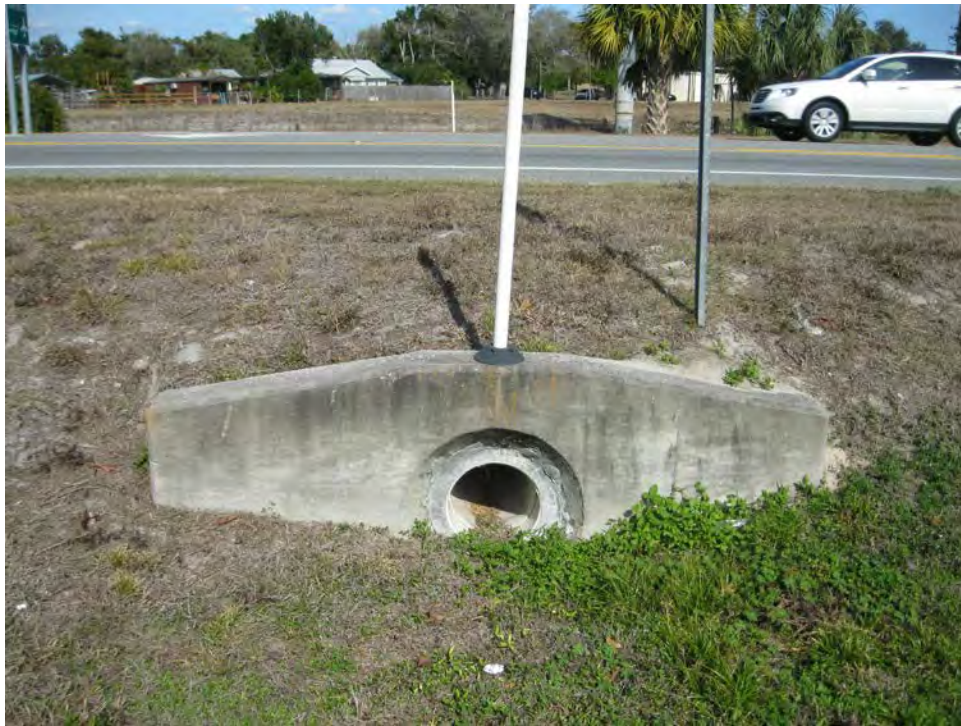
Cross Drain No. 9 – Looking North
