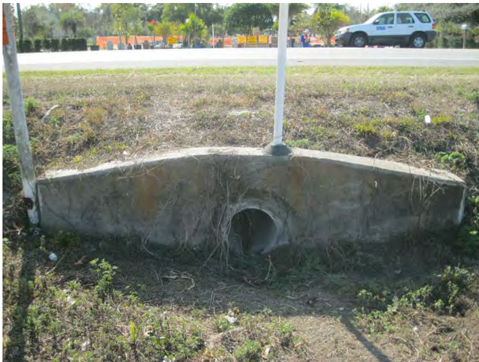
Cross Drain No. 9 – Looking South
