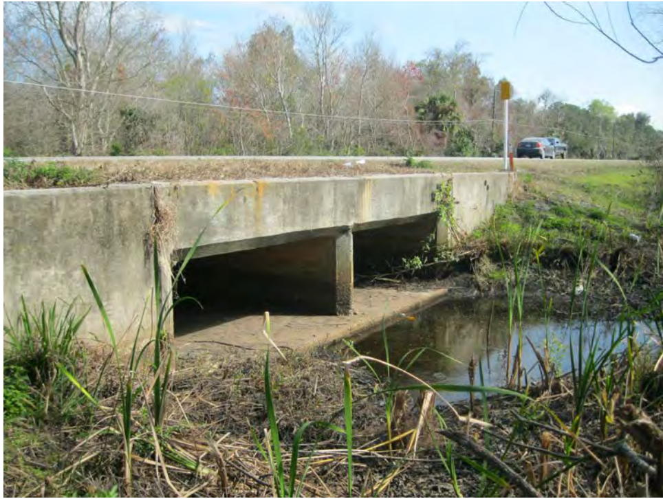
Cross Drain No. 4 – Looking North
