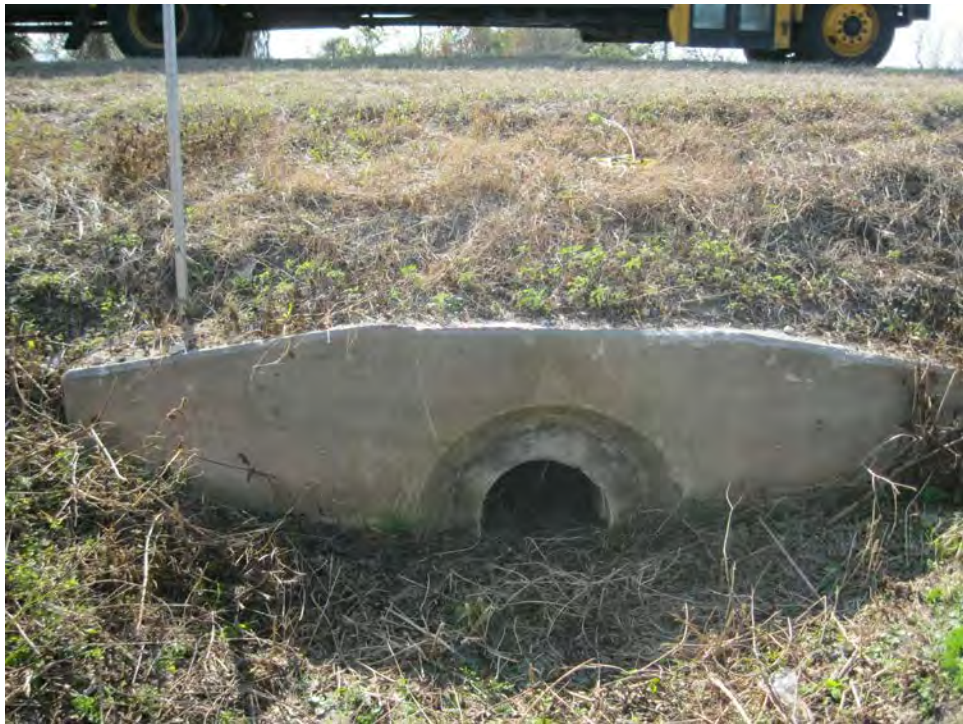
Cross Drain No. 7 – Looking South
