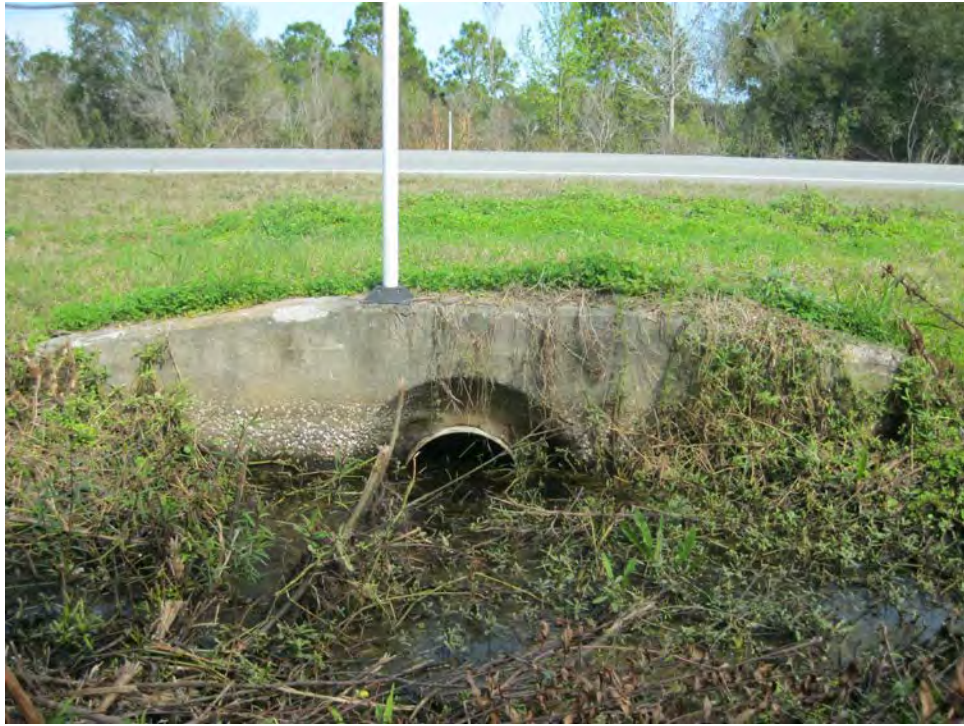
Cross Drain No. 3 – Looking North
