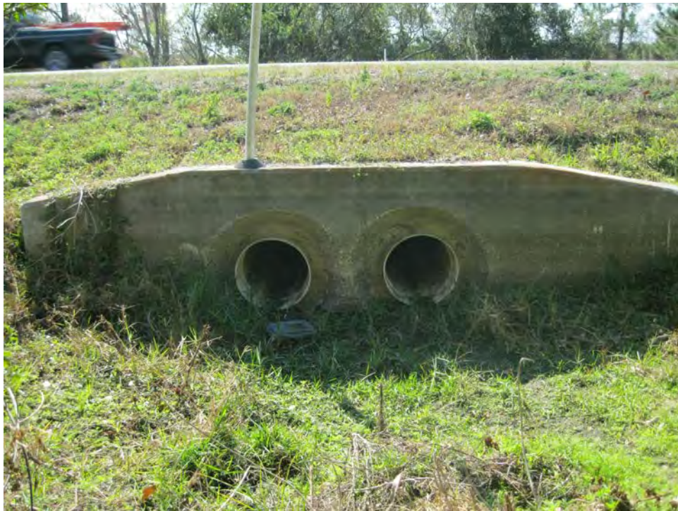
Cross Drain No. 5 – Looking South
