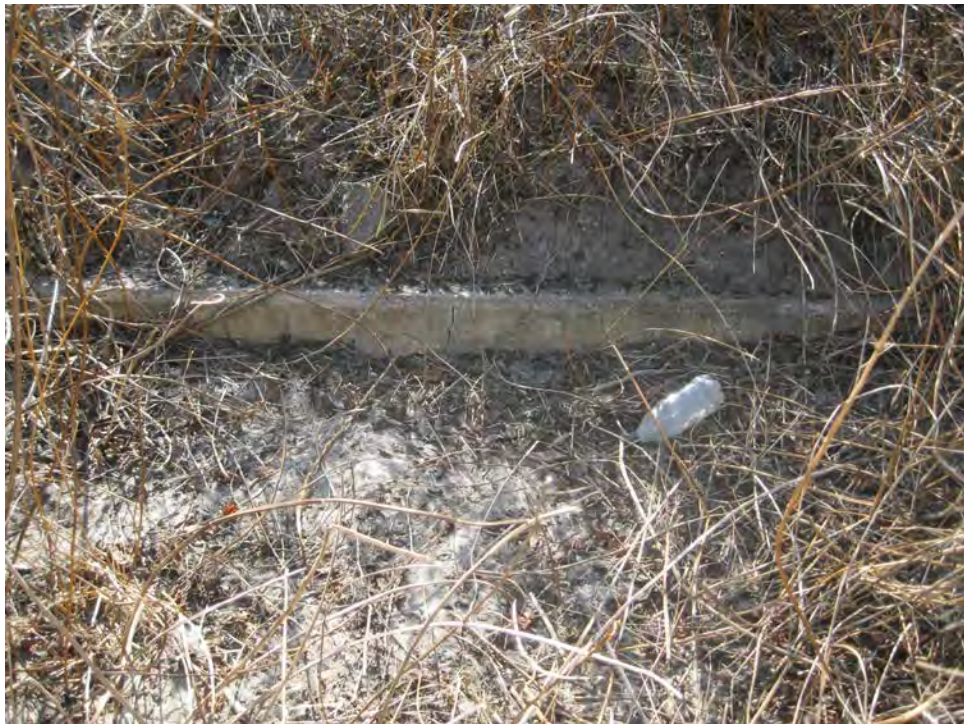
Cross Drain No. 8 – Looking South
