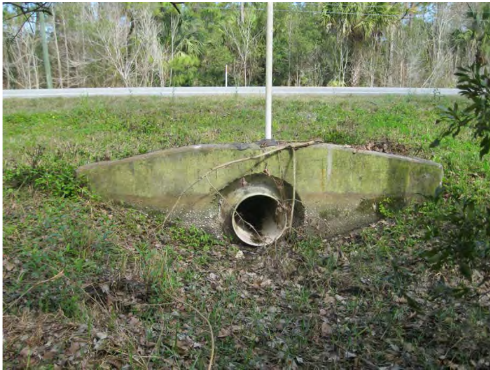
Cross Drain No. 2 – Looking North
