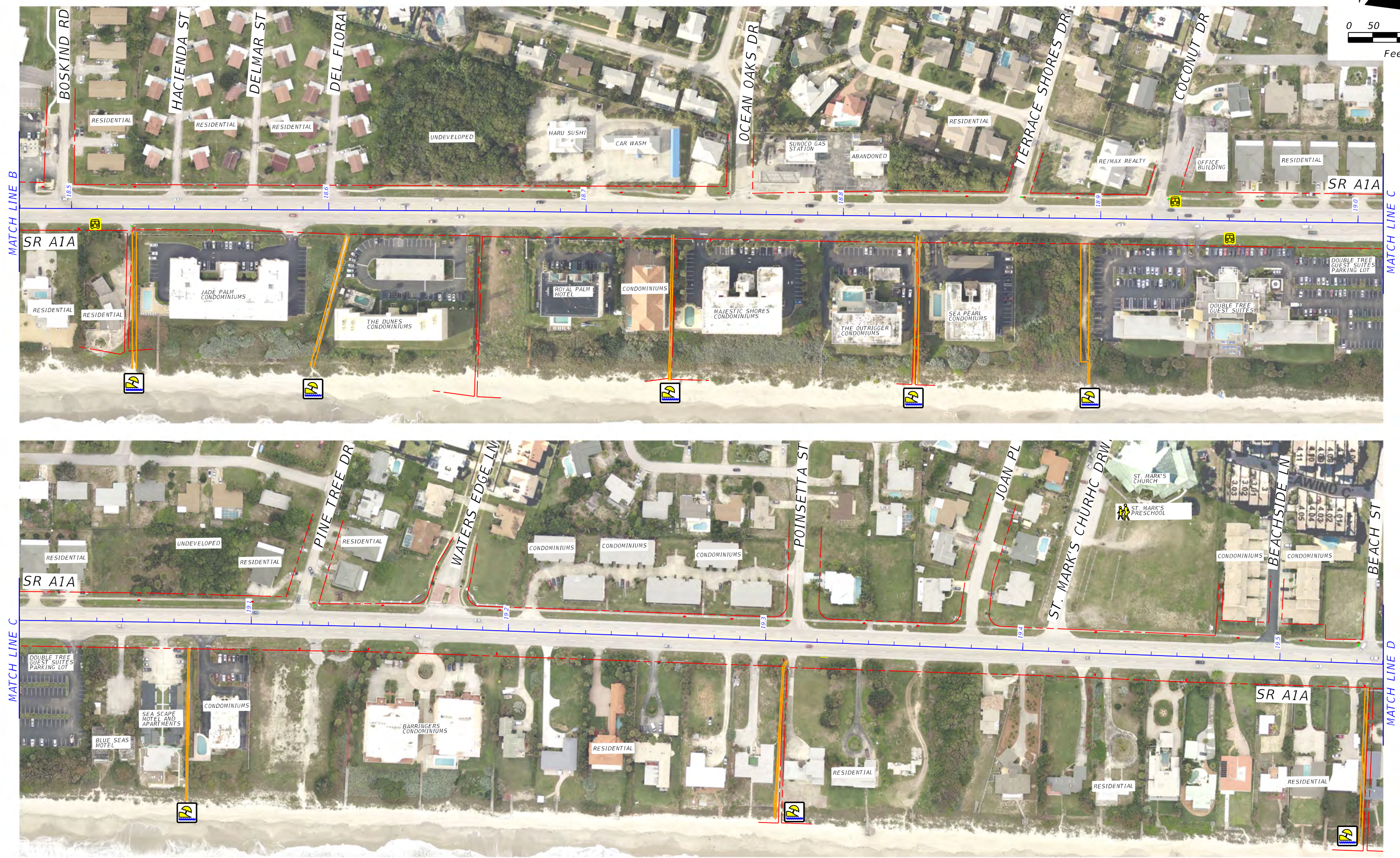
SECTION 70060 - MP 17.536 - MP 20.909 SR A1A FROM US 192 TO SR 518 BREVARD COUNTY - FLORIDA
