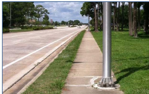
*A street light reduces the usable width of the sidewalk.*
