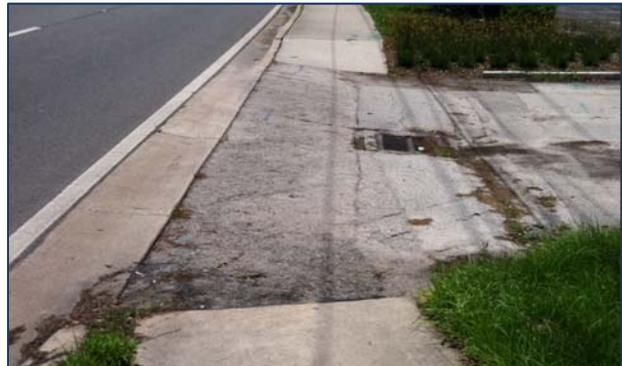
*The ramps at this sidewalk lack truncated domes and the driveway has an uneven surface.*
