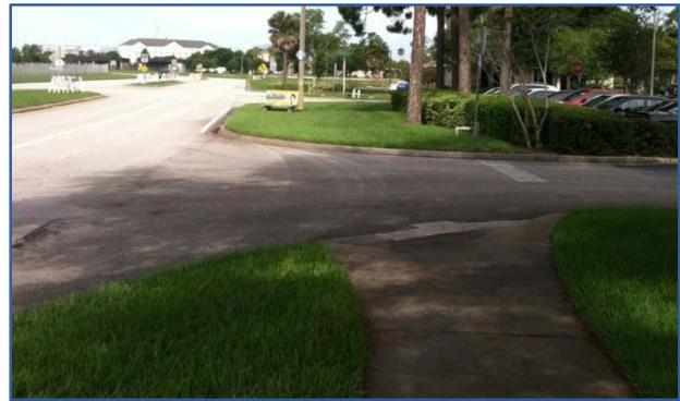
*A non ADA compliant bus stop and sidewalk gap on Richard Petty Blvd at Corsair Dr. The bus stop is located on the utility pole above the bench in the background.*
