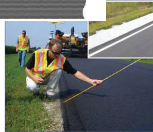
SAFETY EDGE FOR ASPHALT TRAIL
