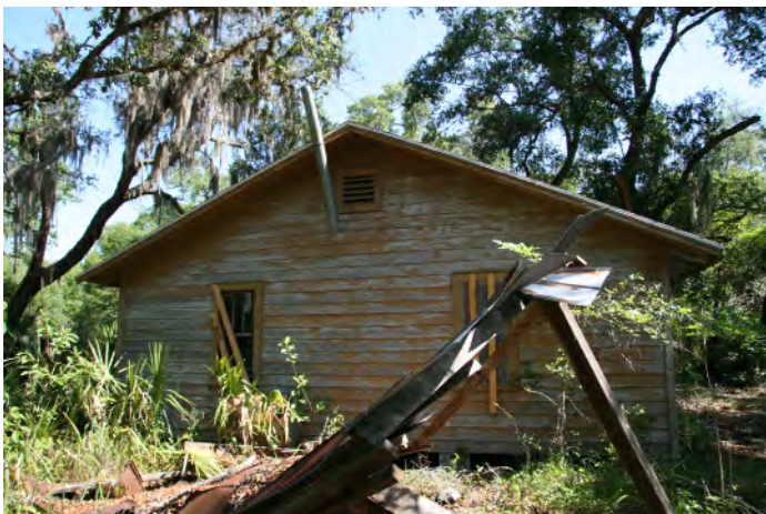
8VO09385_e Facing North
