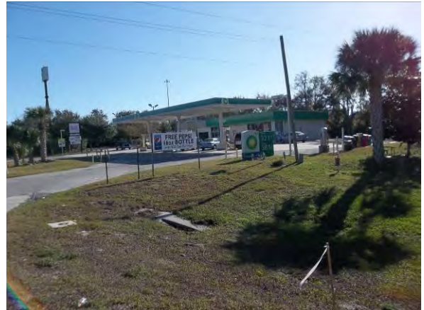
Photo #2 BP Station, 1628 W Granada, Facility #16
