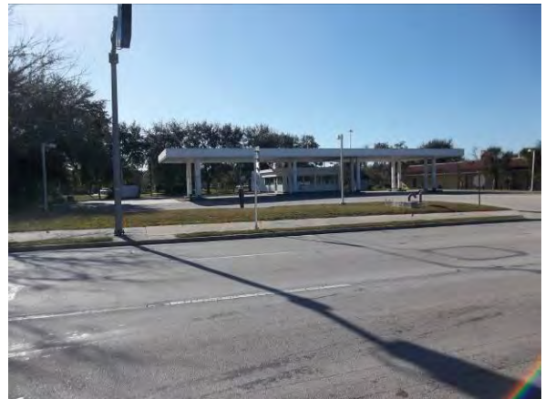
Photo #4 Vacant vehicle fueling station, 1546 W Granada, Facility #20
