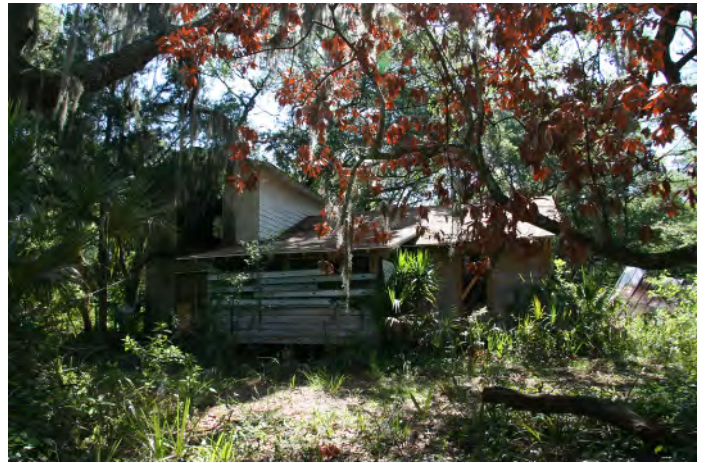
8VO09385_d Facing East
