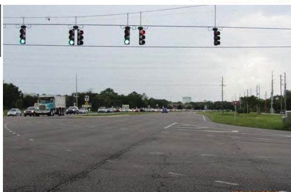
Looking North at SR 536/World Center Drive
