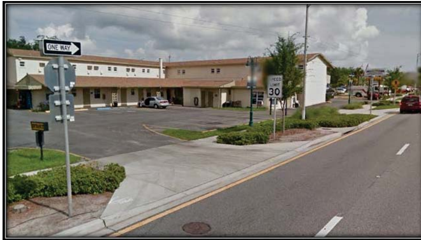
Figure 26: Property with Multiple Driveways
